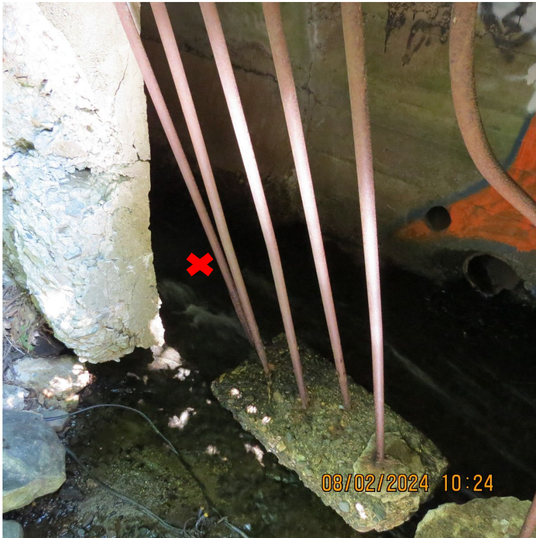
Photo 3: LQ-13A (photo taken 08/02/2023 at approx. 10:24) Stream located near 240 Coburn Ave, discharging into the unnamed stream to Lake Quinsigamond. Sample points are indicated by a red X
