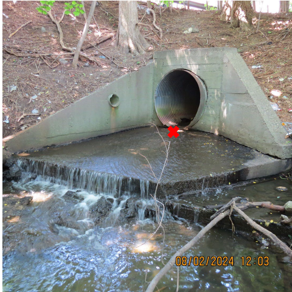
Photo 5: CM-05 (photo taken 08/02/2023 at approx. 12:03) Outfall located near 481 Lincoln Street, discharging into the unnamed stream discharging to Cole Mine Brook. Sample points are indicated by a red X
