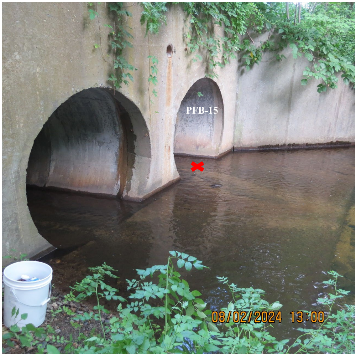
Photo 7: PFB-15(right) (photo taken 08/02/2023 at approx. 13:00) Outfall located near 275 Clark Street, discharging into the unnamed stream discharging to Poor Farm Brook. Sample points are indicated by a red X
