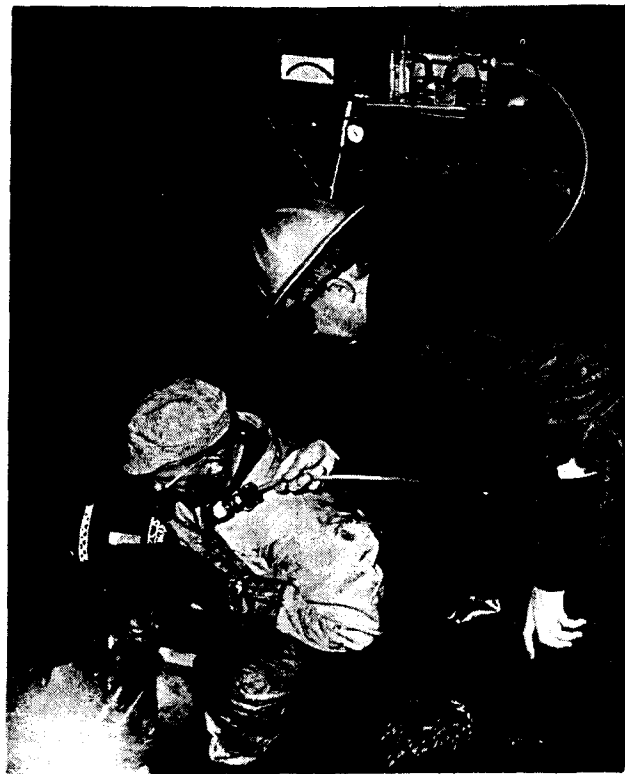
Fig. 6 (left). Welding without ventilation is shown being studied. A sample of fumes taken in the welder's breathing zone was measured at 80 mg per cu. m. Fig. 7 (right) shows same situation but with a downflow general exhaust of 53 fpm average velocity being employed. The fume concentration was reduced to 5 mg per cu. m.
