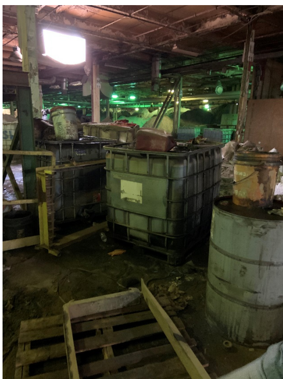
Figure 27: IMG_3096.jpg – Containers of unknown waste in the Keebler Building
