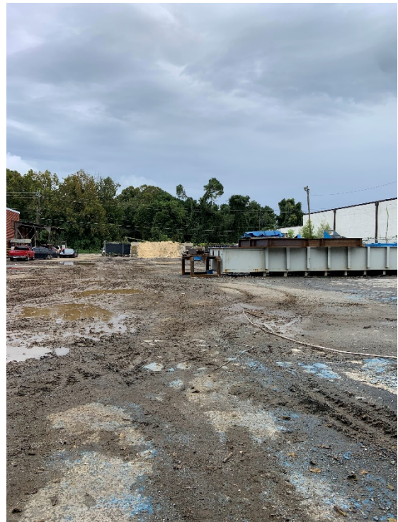
Figure 16: IMG_3085.jpg– Rear of Fabrication Building
