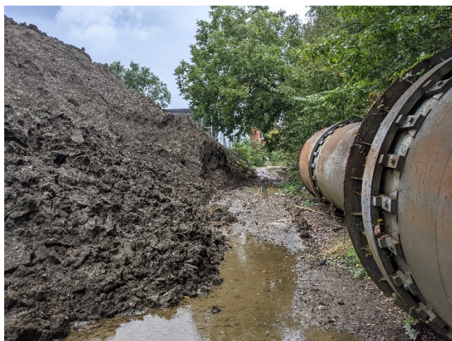
Figure 99: PXL_20211006_181118853.jpg – Rear side of solid waste pile near Outfall 3
