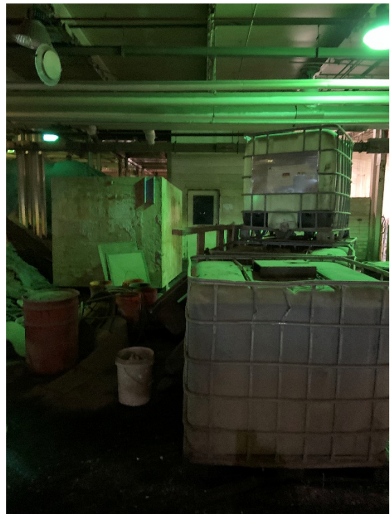
Figure 32: IMG_3101.jpg - Containers of unknown waste in the Keebler Building
