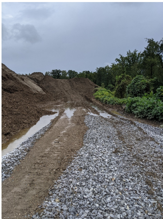
Figure 110: PXL_20211006_183813827.jpg – Solid Waste Pile/Landfill Laydown Yard
