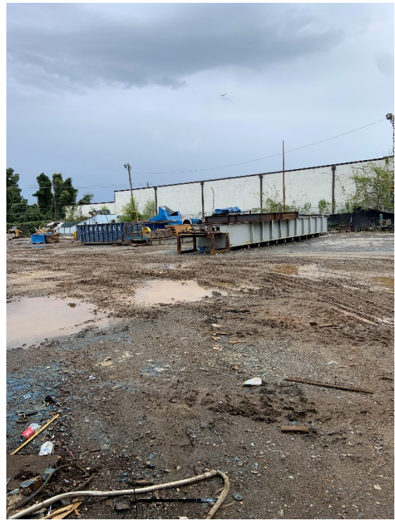
Figure 14: IMG_3083.jpg – Rear of Fabrication Building
