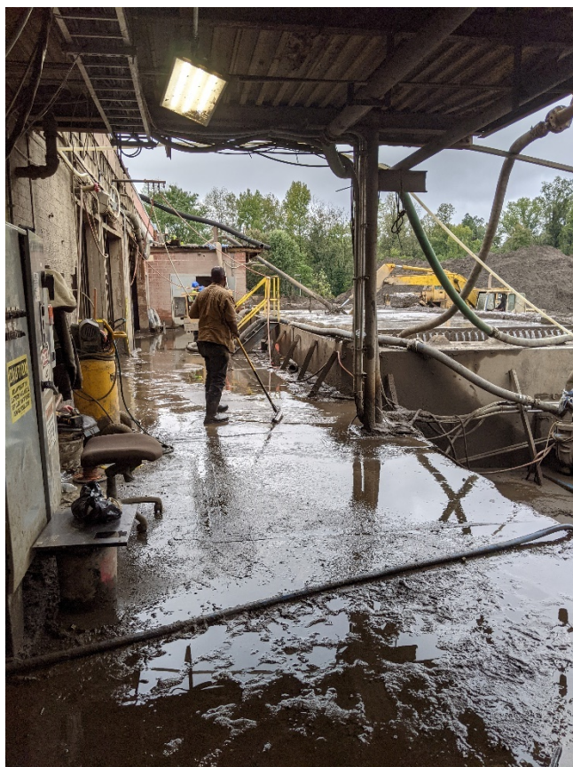
Figure 79: PXL_20211006_151149845.jpg – Wastewater Treatment Area
