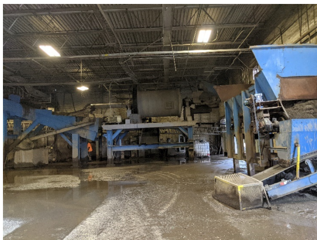
Figure 52: PXL_20211006_142355136.jpg – Processing in White Building
