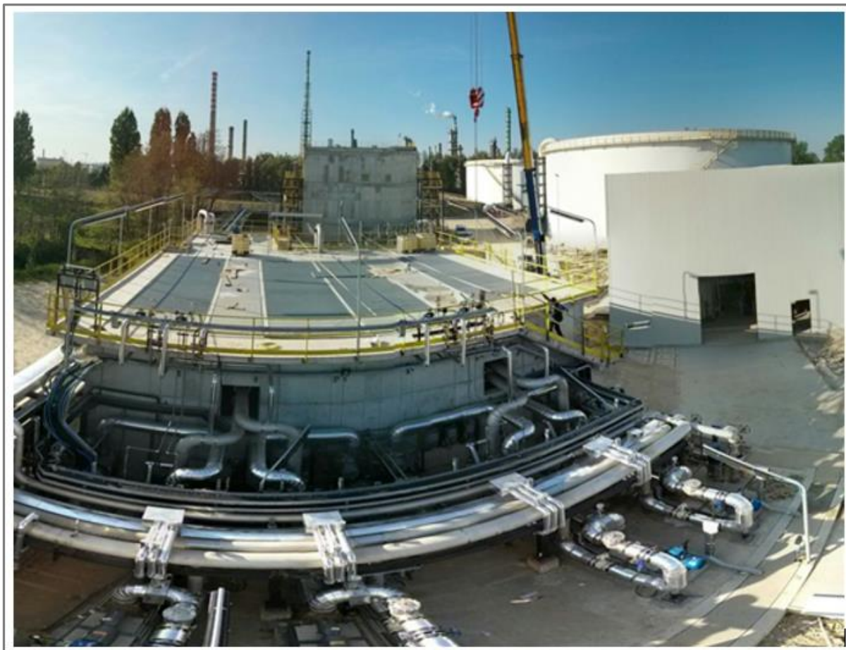
FIGURE 22: INFRASTRUCTURE PICTURE OF THE INDUSTRIAL PLANT IN ITALY.
