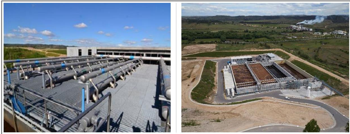
FIGURE 21: INFRASTRUCTURE PICTURE OF INDUSTRIAL WW TREATMENT PLANT IN PORTUGAL.
