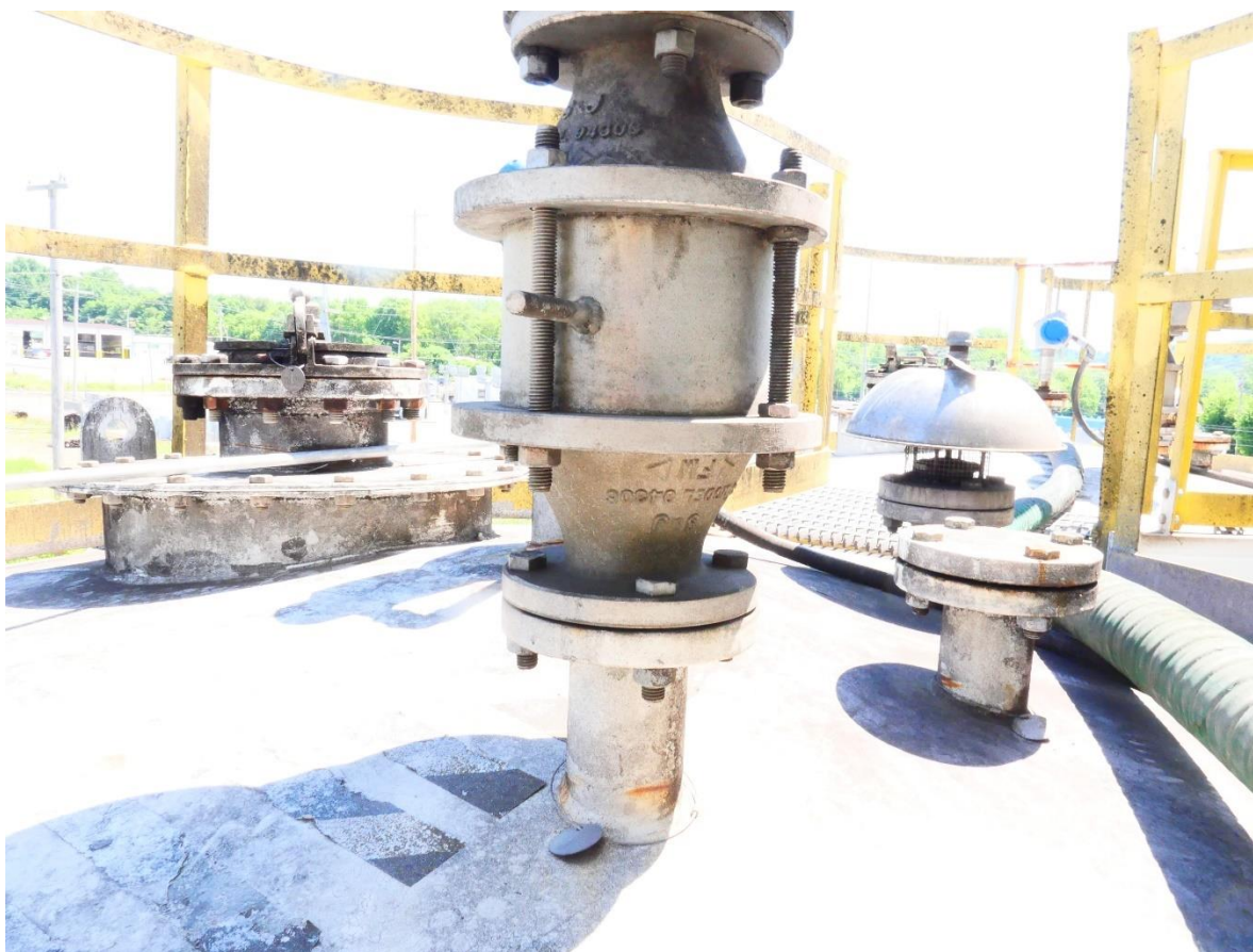
Photo 12: Tank System 2 – Roof Top
