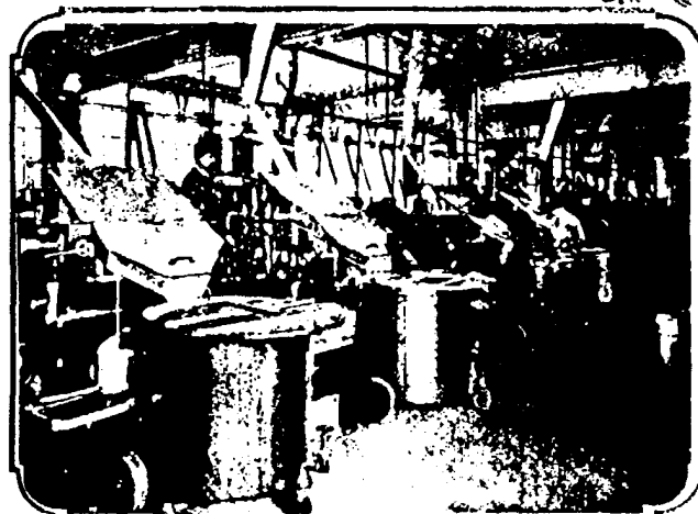
Another Interior View showing a Battery of the most Modern Type of Paint Grinding Machines.
