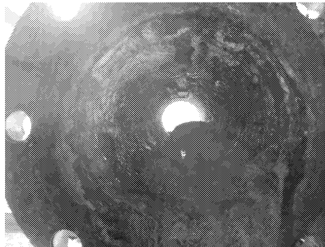
Build Up on Walls of Contact Chamber
