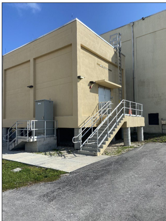
Photo 1: New headworks building.
