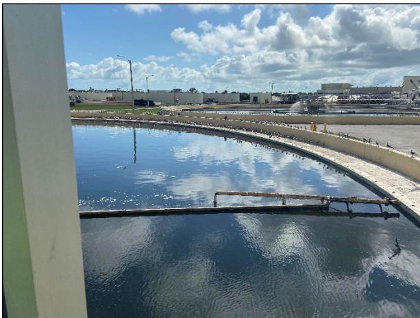
Photo 9: Plant 2 secondary clarifier.
