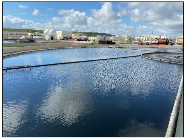
Photo 6: Plant 1 secondary clarifier.
