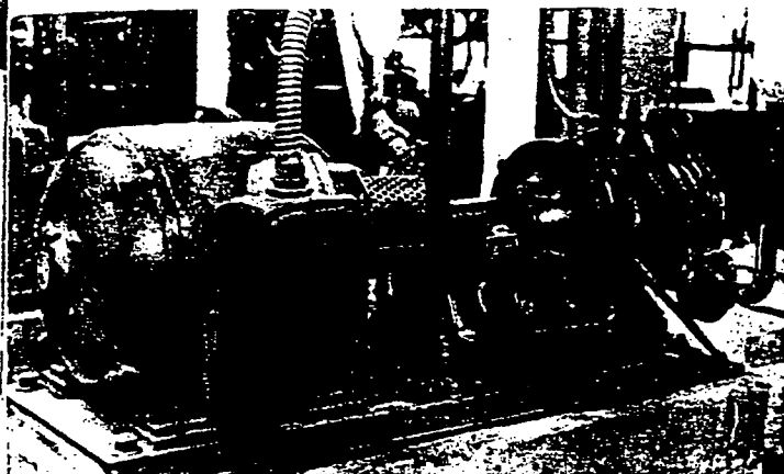
Left and below—Three Elliott Crocker-Wheeler 25-hp, 3600-rpm motors driving desuperheater water pumps.
