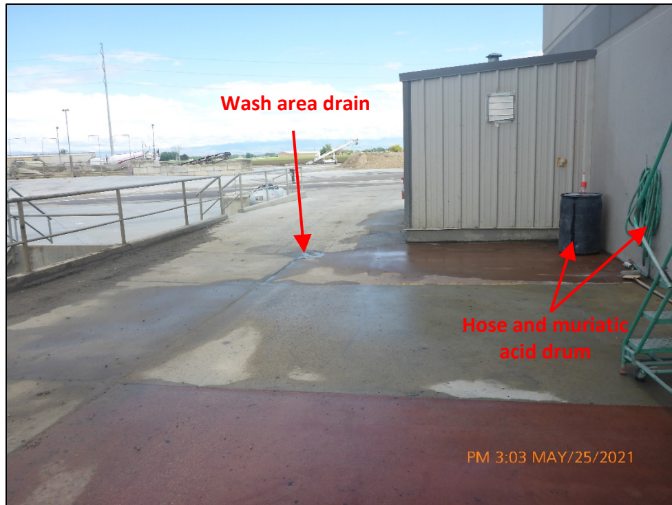
Photograph 9. View, facing east, of an outdoor wash area located north of the maintenance building. Note the hose and 55-gallon drum of muriatic acid. This wash drain flows to the onsite subsurface infiltration structure located north of the maintenance building.
