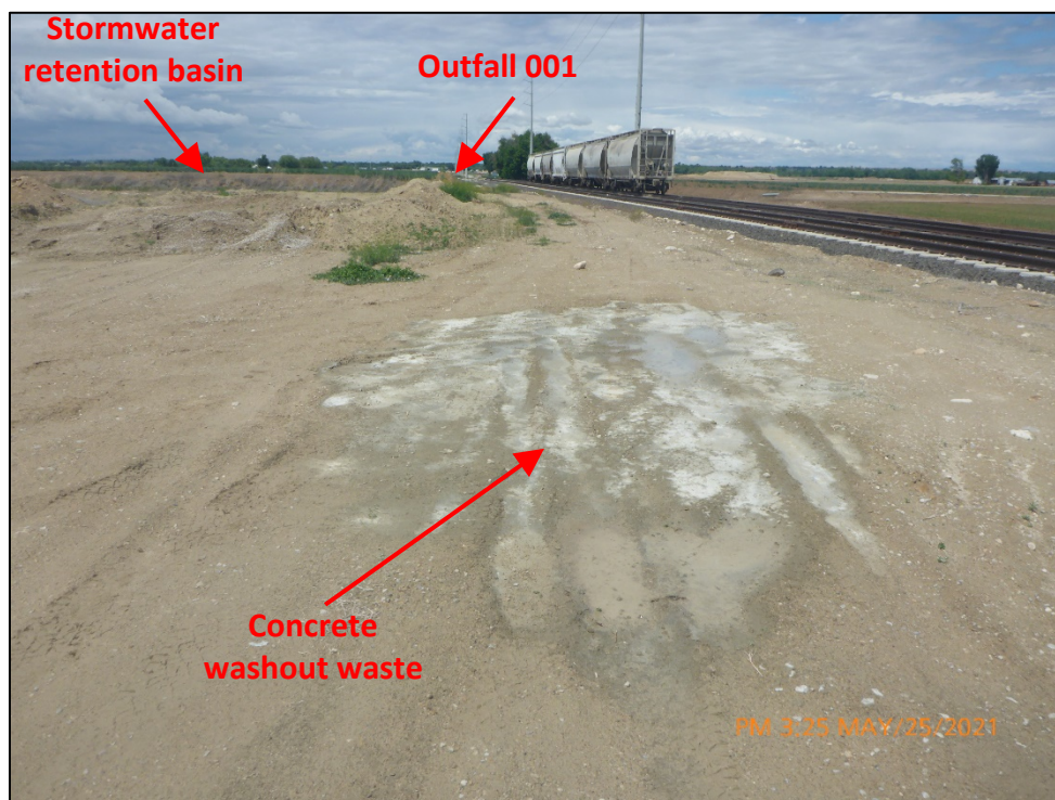
Photograph 14. View, facing north, of the concrete washout waste on the ground surface in the northeastern portion of the Facility, upgradient of the stormwater retention basin and Outfall 001.
