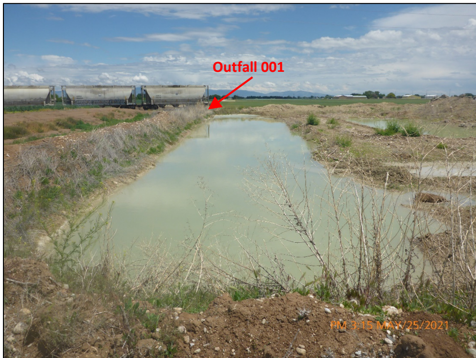
Photograph 2. View, facing east, of the stormwater retention basin in the northern corner of the Facility. Outfall 001 is located at the basin's spillway on the northeast corner.
