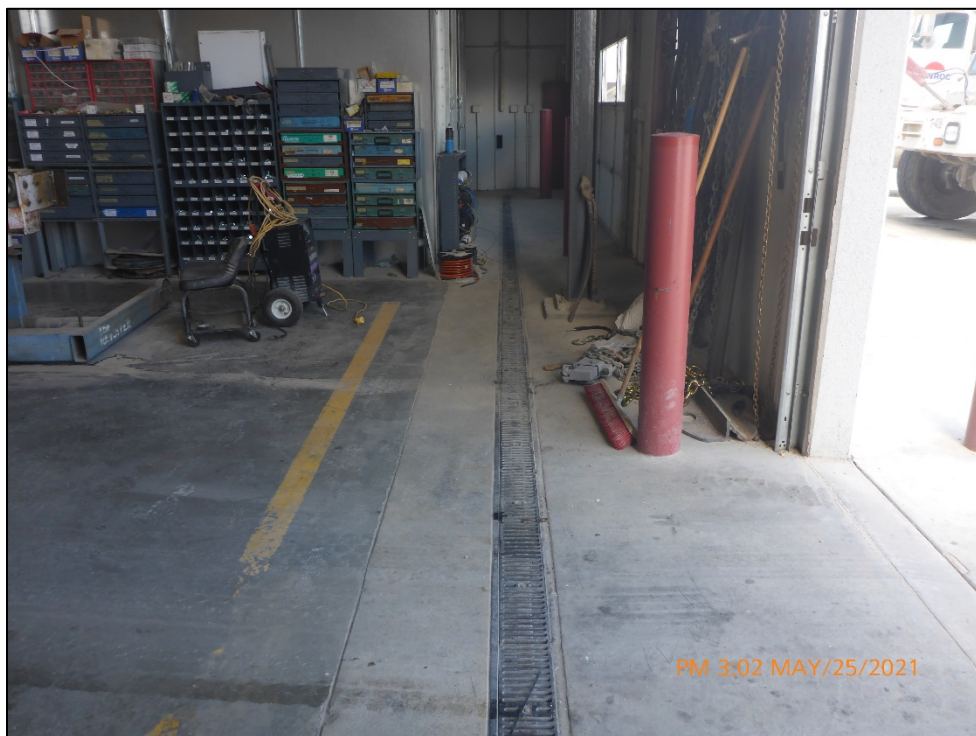
Photograph 8. View, facing north inside the maintenance building, of a trench drain that flows to an onsite subsurface infiltration structure located north of the maintenance building and adjacent fuel island.
