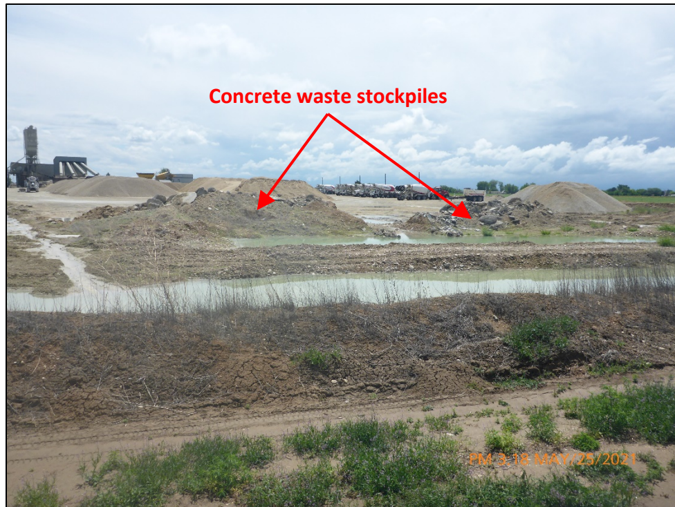
Photograph 5. View, facing southwest, of concrete waste stockpiles on the south side of the stormwater retention basin (between the two inlets to the basin) shown in Photographs 3 and 4.
