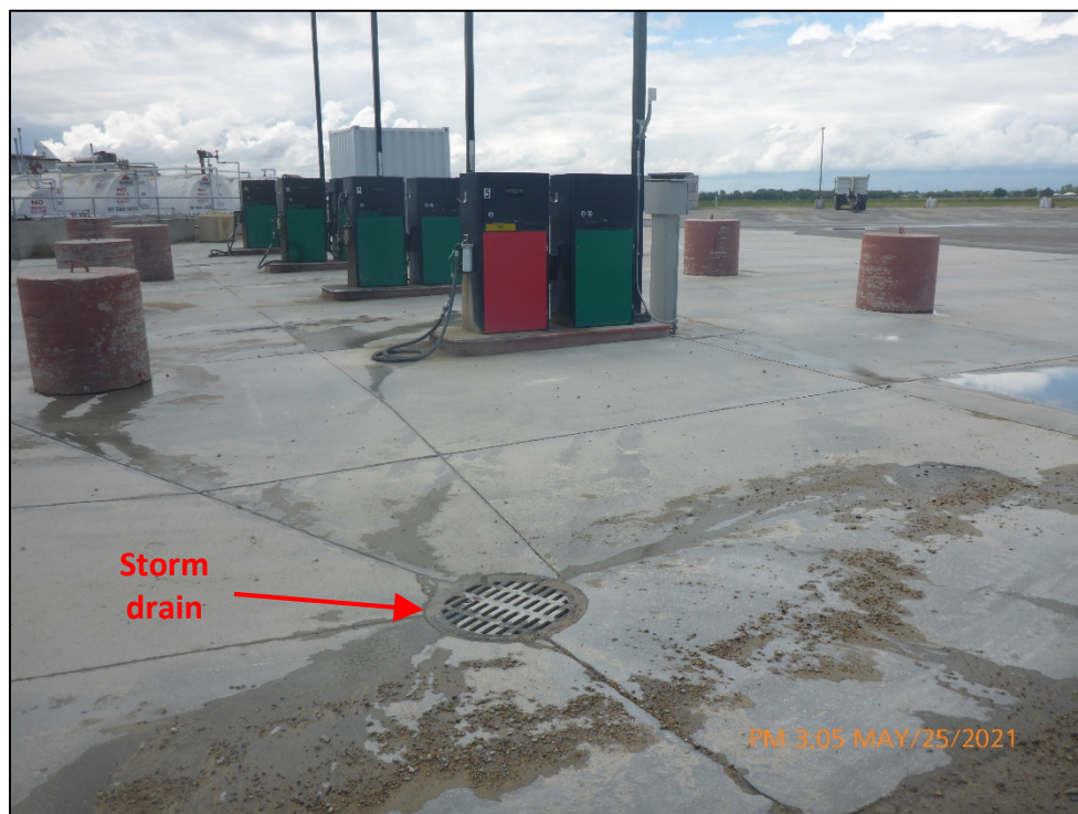
Photograph 10. View, facing west, of a storm drain near the fuel island that is north of the maintenance building and outdoor wash area shown in Photographs 8 and 9. Mr. Henderson confirmed that this storm drain is connected to the onsite subsurface infiltration structure.
