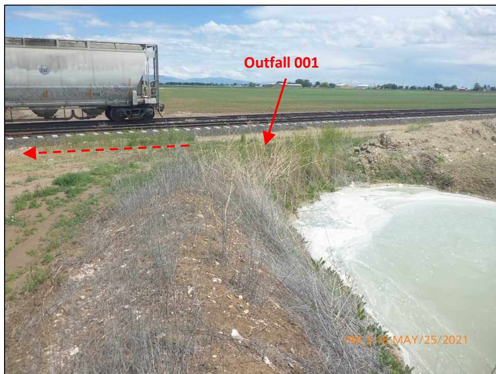
Photograph 6. View of the overflow point of the stormwater retention basin, noted as Outfall 001. Red dotted arrow indicates flow direction from Outfall 001 to the Lower Fivemile Drain.
