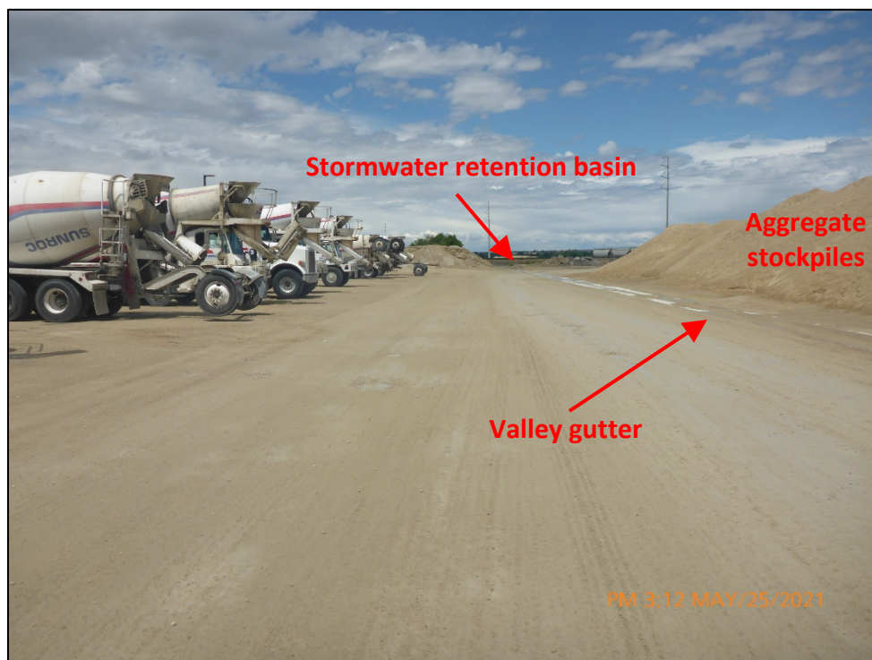
Photograph 12. View, facing north, of the valley gutter that flows north to the stormwater retention basin, located along the west side of the Facility between the concrete truck parking area and aggregate stockpiles.
