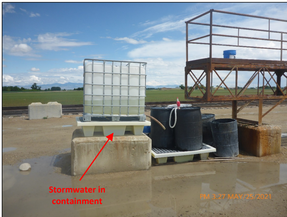
Photograph 16. View, facing east, of concrete stripping chemicals stored at the truck wash rack shown in Photograph 15. Note this wash rack is not identified on the SWPPP site map. Due to recent heavy precipitation, the secondary containment units were full of stormwater.
