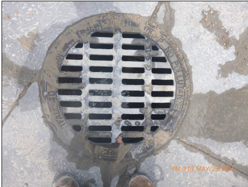
Photograph 11. Close-up view of the storm drain shown in Photograph 10. This grate is casted with the message "Outfall To Stream. Dump No Pollution".
