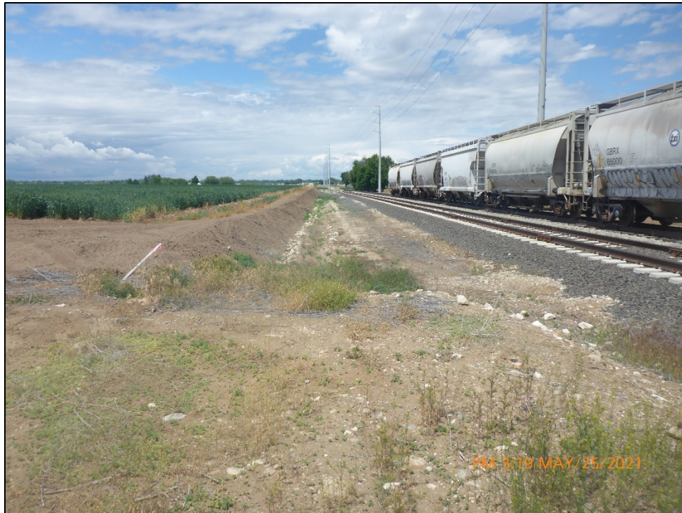
Photograph 7. View, facing north from Outfall 001, of the stormwater flow pathway along the railroad right-of-way from Outfall 001 toward the Lower Fivemile Drain.
