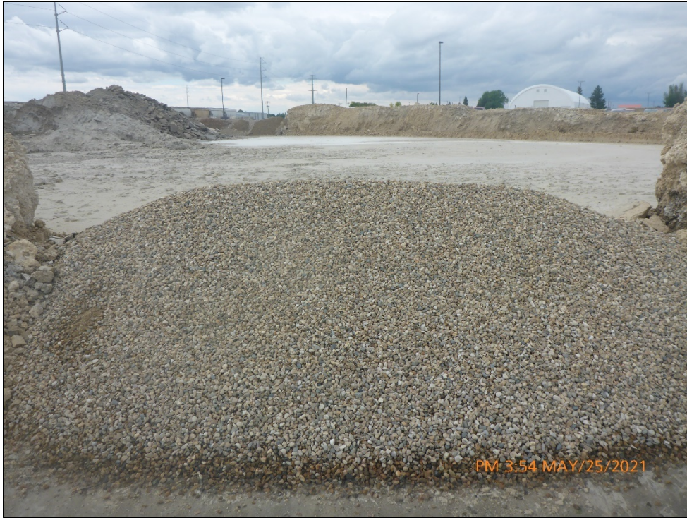
Photograph 19. View, facing south, of the aggregate and waste concrete drying basin south of the wash water recycling system shown in Photograph 18. Settled solids from the wash water recycling system settling bays, as well as other wet concrete waste, is allowed to dry and harden in this basin.
