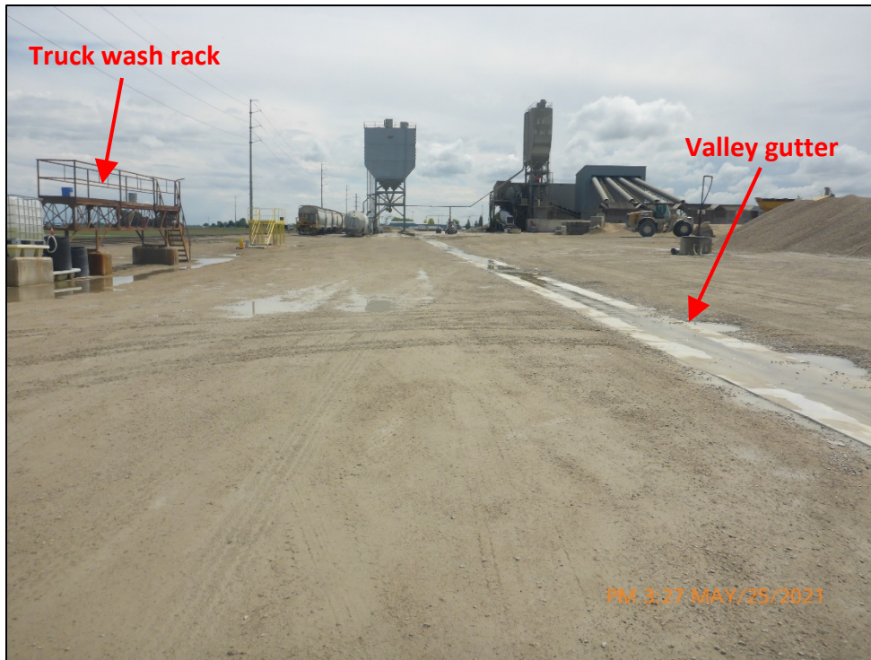
Photograph 15. View, facing south, of an uncovered truck wash rack located in the northeastern portion of the Facility. Wash water from this wash rack would appear to flow over the gravel surface, into the valley gutter, and subsequently into the stormwater retention basin.
