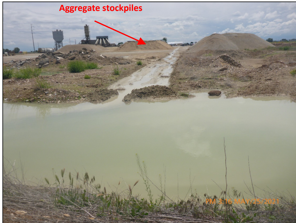
Photograph 3. View, facing south, of the inlet on the west side of the stormwater retention basin. A valley gutter that runs north between the concrete truck parking area and aggregate stockpiles enters the basin at this location.
