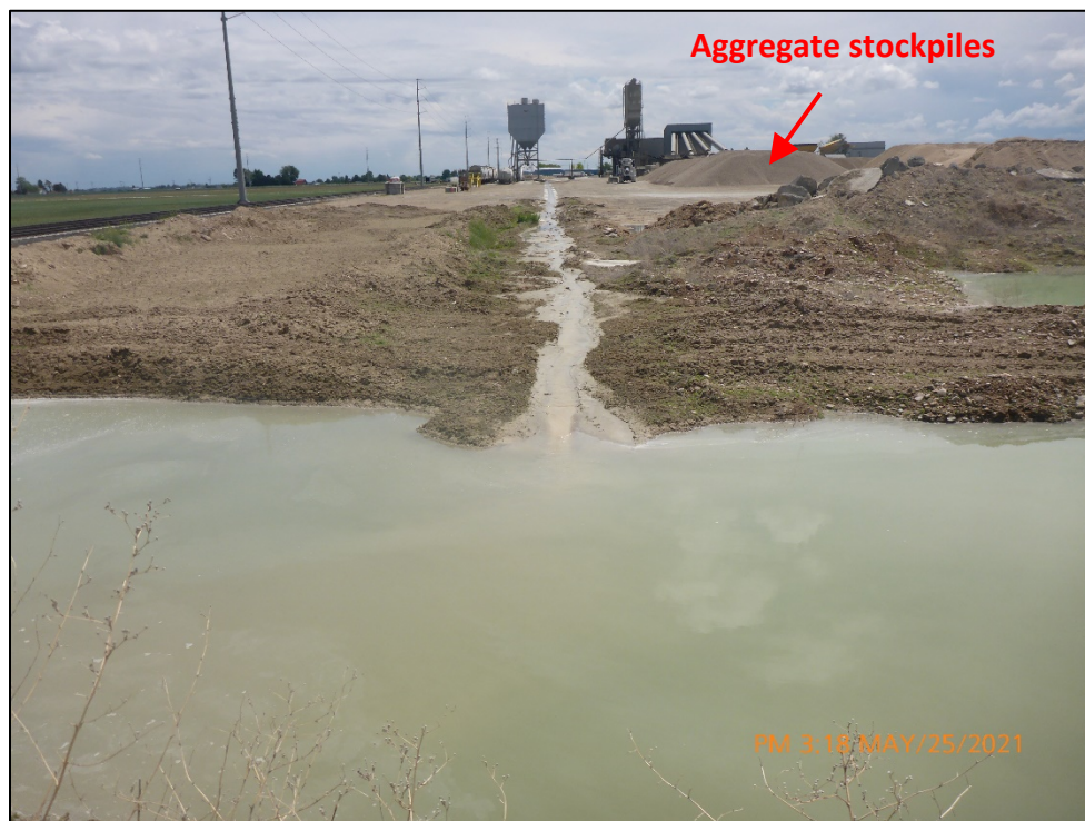
Photograph 4. View, facing south, of the inlet on the east side of the stormwater retention basin. A valley gutter that runs north between the aggregate stockpiles and the Facility's eastern perimeter enters the basin at this location.
