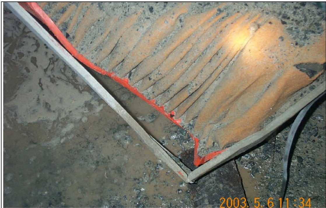
Condition of Dynavane Primary Filter – X days after installation.
