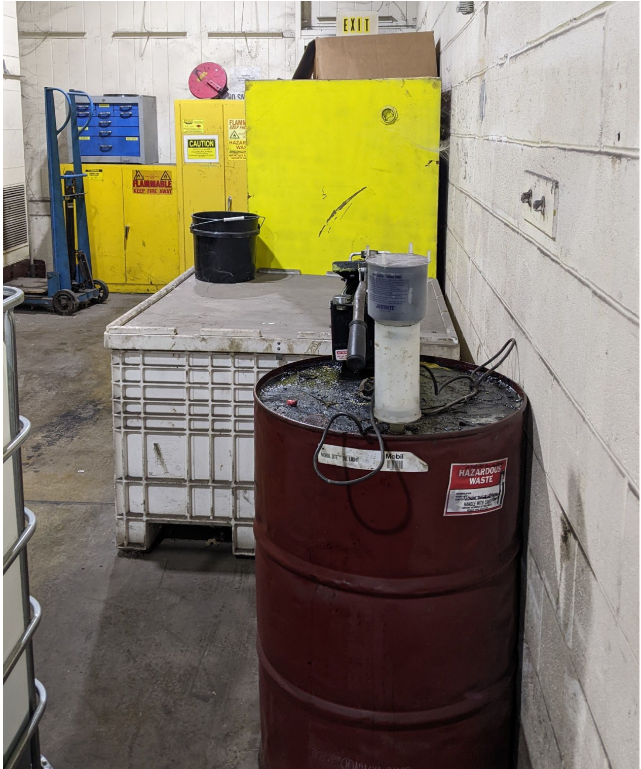
Photo #4: View of the relocated satellite container in the Waste Accumulation Room.
