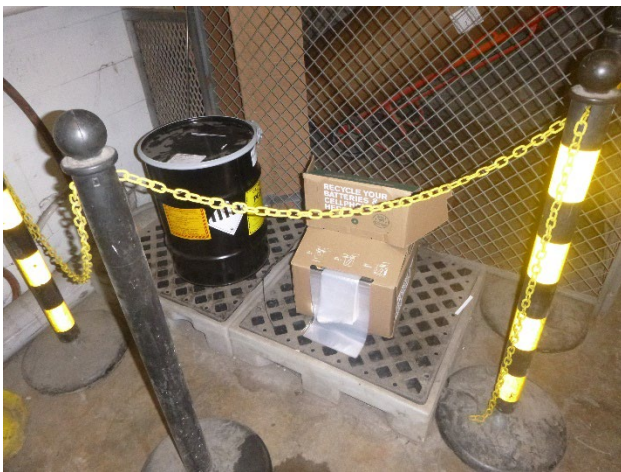
Photo 8: Coal Plant Powerhouse.
