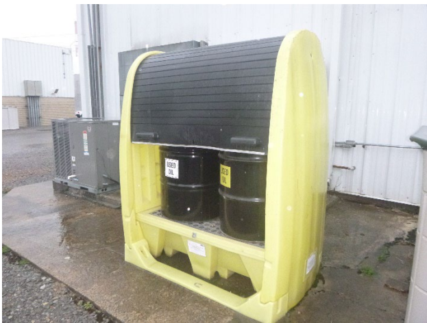
Photo 2: Combustion Turbine Area.
