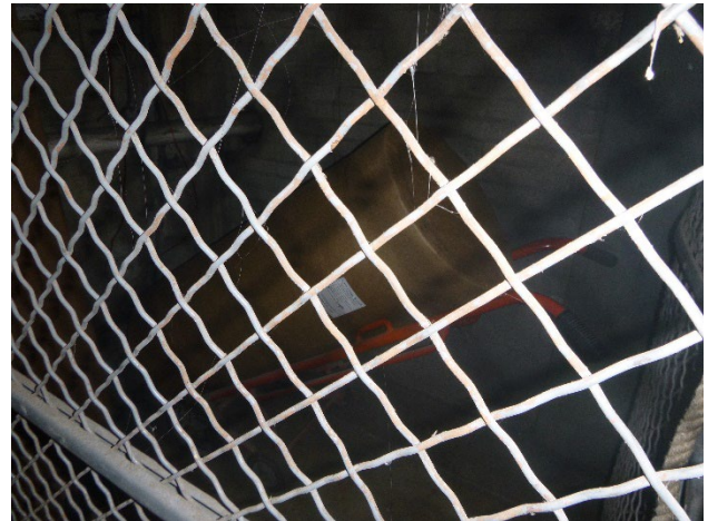
Photo 6: Coal Plant Powerhouse.
