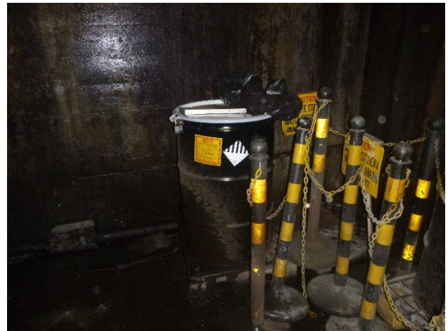
Photo 10: Coal Plant Powerhouse .
