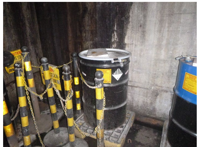
Photo 11: Coal Plant Powerhouse .
