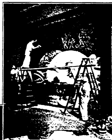
(Left) Wall coated with white lead-varnish paste. (Right) Rolling the mural smooth over the wall coated with white lead and varnish. Mr. Charles Knight, who painted the mural, is viewing the work. (Below) New Hayden Planetarium, New York City. Trowbridge and Livingston, Architects.
