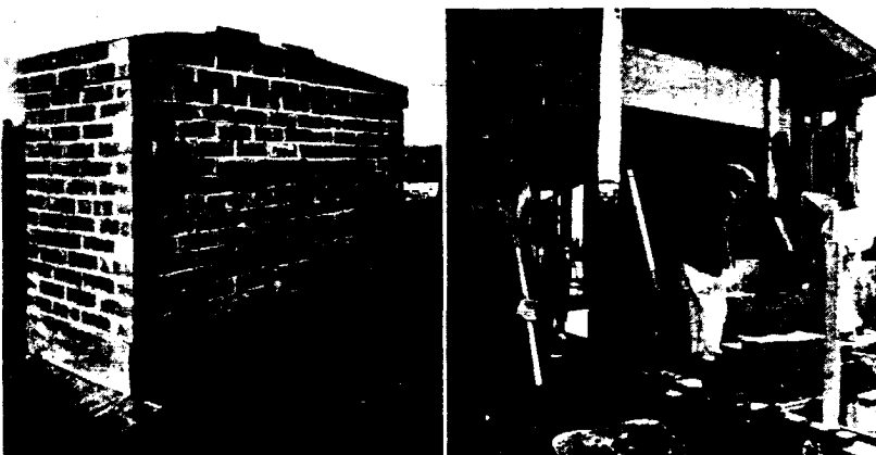
Above left, lead chimney flashing is installed in the usual manner. The lead slag stop can just be seen at the left where it dies into the chimney flashing. Above right, erecting the chimney. The joint between the brick chimney and shingled wall is flashed with strips of lead, installed in short sections and overlapped. Below, the lead flashing and fascia band for the composition deck
