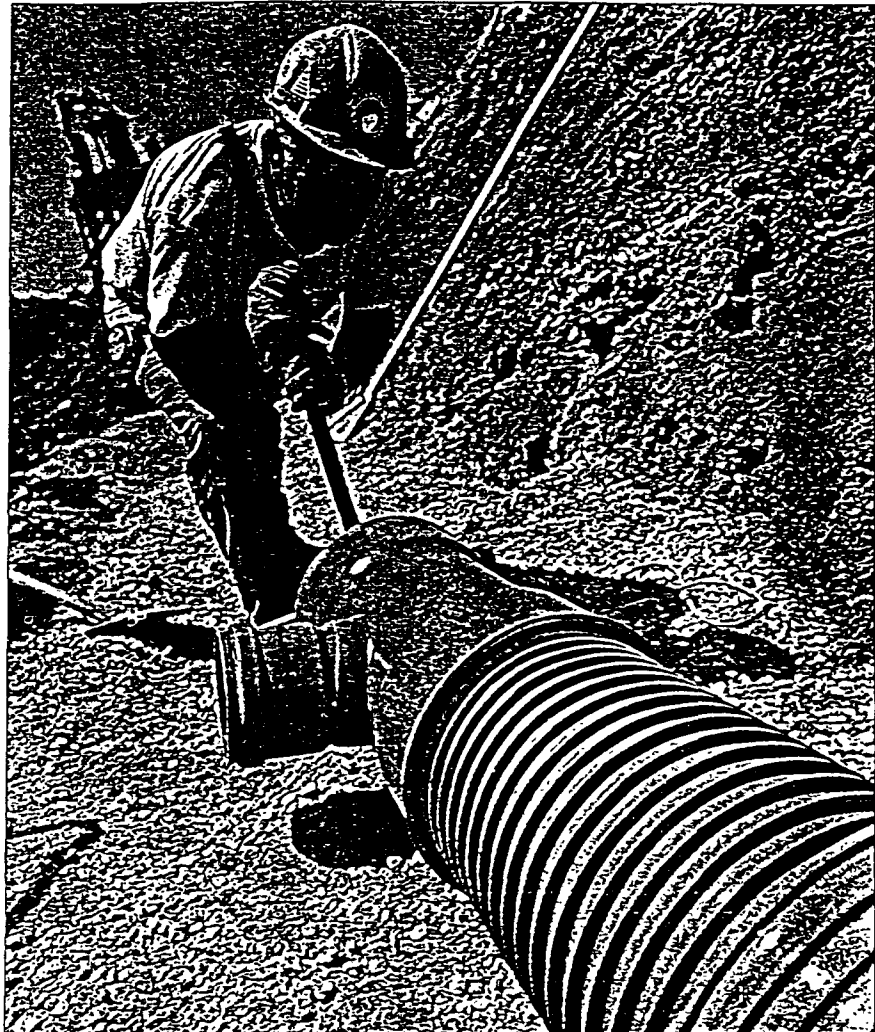
An unidentified worker installs a PVC Ultra-Rib sewer pipe with a PVC fitting. This type of PVC pipe complies with ASTM Standard F794.
