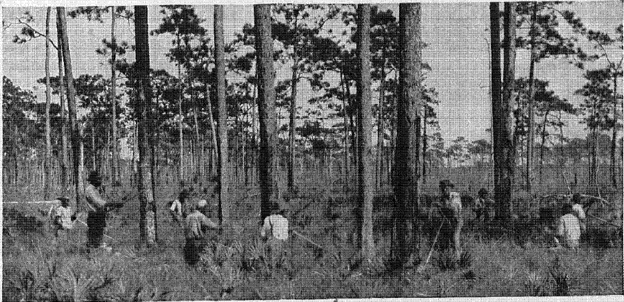
Land clearing with dynamite near Bradentown, Florida. The explosive lifted the trees out bodily. Tractors and grubbing plows did the rest
