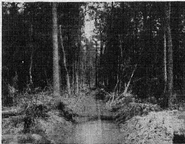
Ditch blasted through cypress and gum swamp at Bamberg, South Carolina, by the U. S. Public Health Service in a malaria-control campaign. Top width, 10 feet; bottom, 6 feet; depth, 4 feet. The right of way was not cleared and the ditch was not trimmed after the blast.
