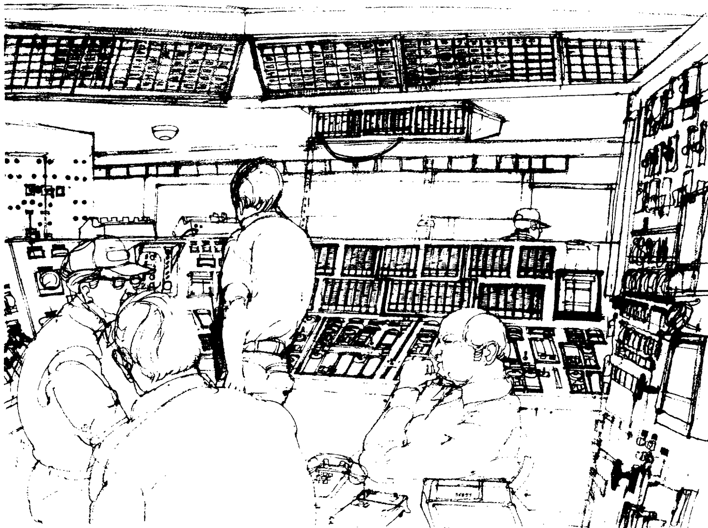
This control room of a typical utility power plant shows how Panalarm® industrial annunciators are installed in the ceiling panel.
