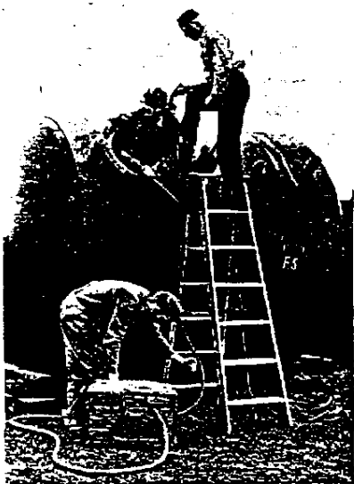
Figure 6. Although this tank has been cleaned and purged of gas, the workmen are equipped for any emergency. (See paragraphs 24 and 40.)
