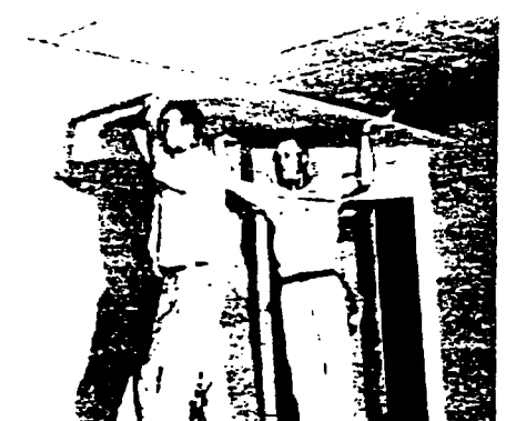
CEMENT IS APPLIED to face layer wallboard to a thickness of 1/4 in. While still wet, face board is then applied and nailed to the joists.
