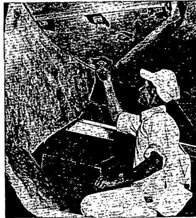
One of many fast methods for Microlite application is with Stic-Klips, as illustrated above.
