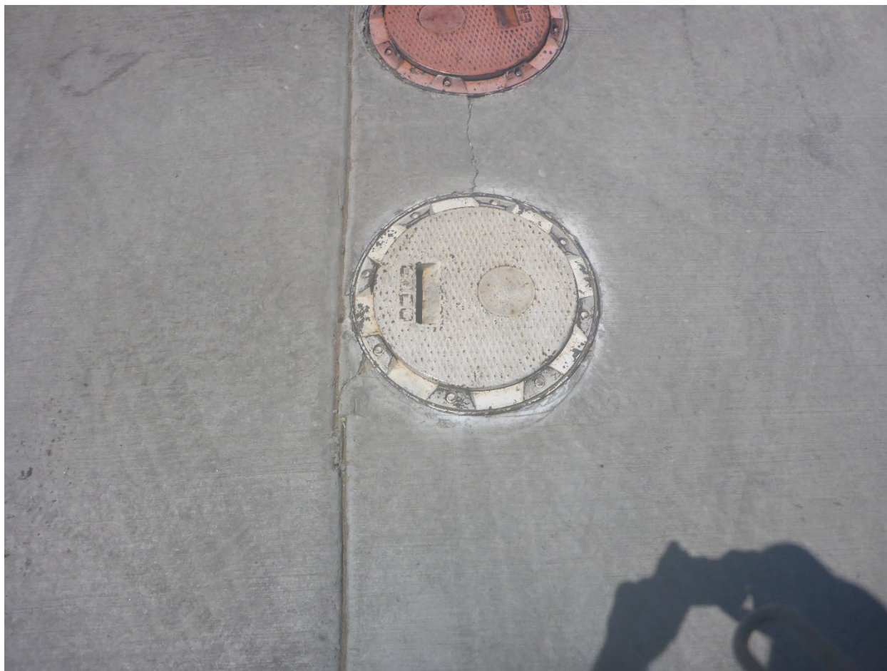
Location Photo – Tank 2B Unleaded
