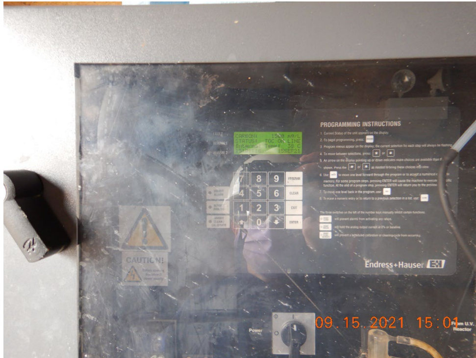
CWA Photo 1. View of the KSR1 TOC analyzer, which read 1,500 mg/l (ppm) at the time of the inspection.
