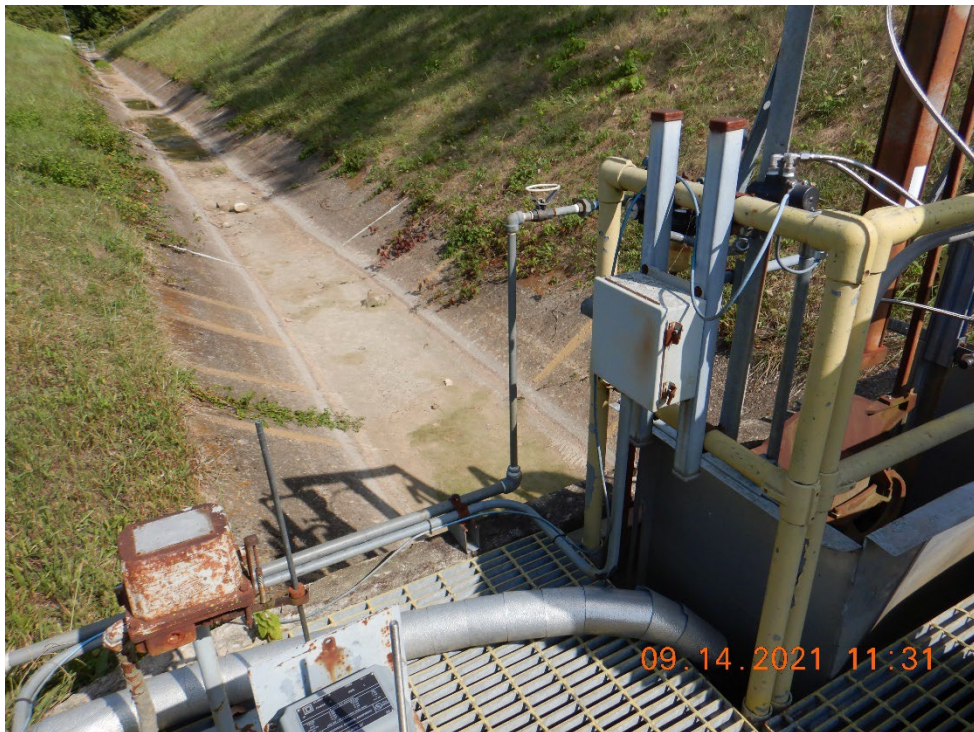
CWA Photo 18. View, facing North, towards Outfall 001, of the concrete ditch used to convey stormwater and NCCW to Outfall 001. Flow was not sufficient to reach Outfall 001 at the time of the inspection.
