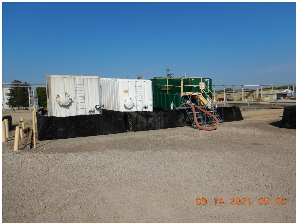
CWA Photo 8. View of the frac tanks being used for intermediate waste storage prior to disposal in the North Lagoon or off site.
