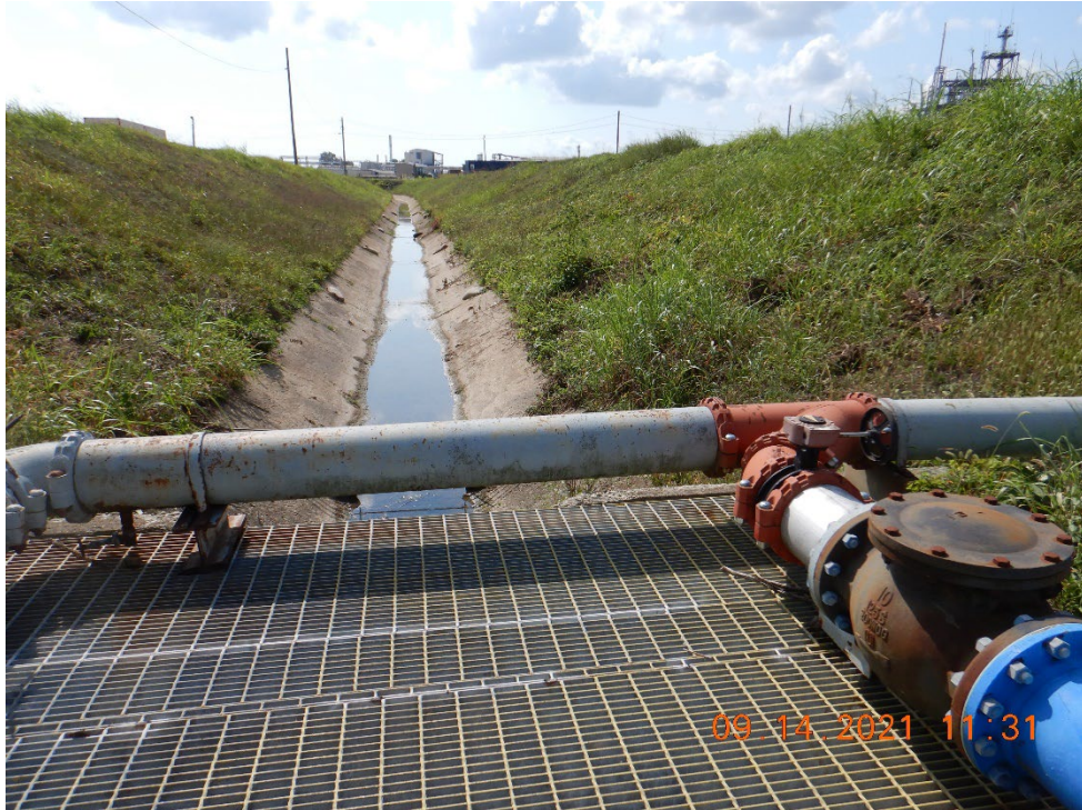
CWA Photo 17. View, facing south, away from Outfall 001, of the concrete ditch used to convey stormwater and NCCW to Outfall 001.
