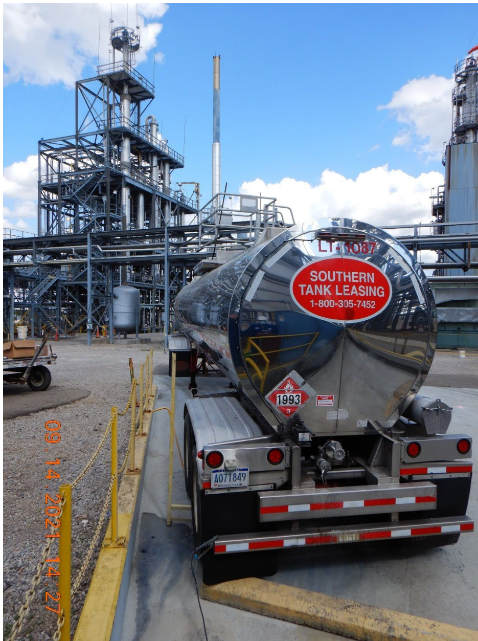
RCRA Photo 14. A view of the 5,000-gallon tanker trailer LT-1087 that is used to accumulate hazardous pyridine and acetone waste. The tanker trailer acts as a less-than-90-day accumulation container located in the Vespel process area.
