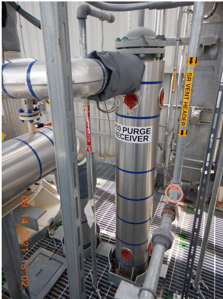
RCRA Photo 5. View of the P-20 purge receiver unit which is used in conjunction with the Kapton solvent recovery unit. The P-20 purge receiver is fed directly to the 5,000-gallon hazardous waste tank shown in Photo 8.
