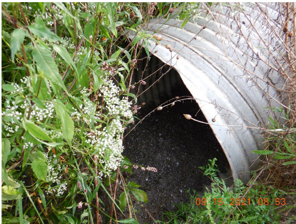
CWA Photo 20. View of stormwater Outfall 003, which was not discharging at the time of the inspection.
