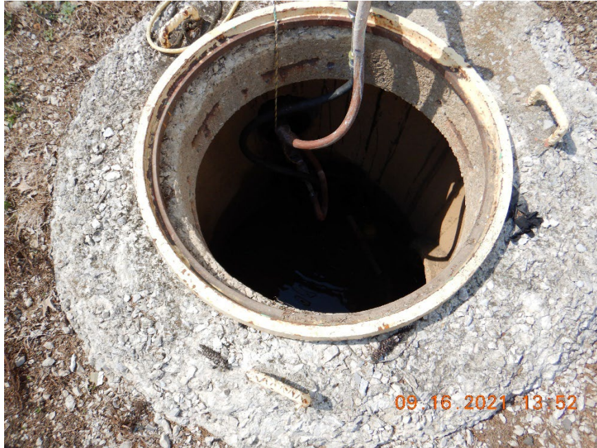
CWA 37. View of the K1 process sewer manhole, near which the Field Blank was transferred.
