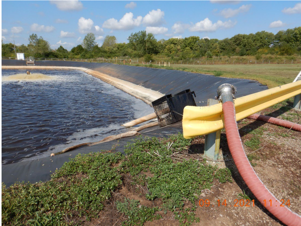
CWA Photo 9. View of the hose used to transfer high organics concentration wastewater, collected by vacuum trucks such as those used at the frac tanks, to the North Lagoon.
