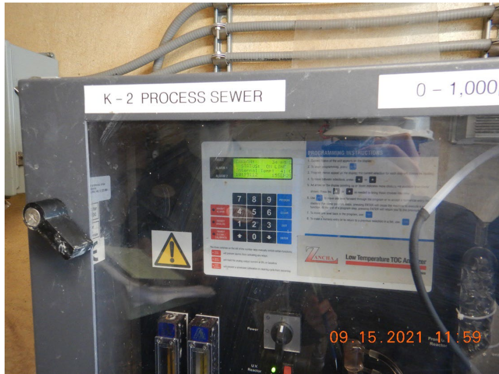
CWA Photo 5. View of the K2 TOC analyzer, which read 34 mg/l (ppm) at the time of the inspection on 9/15/2021. The time reading on this analyzer was off by 1 hour and 40 minutes.
