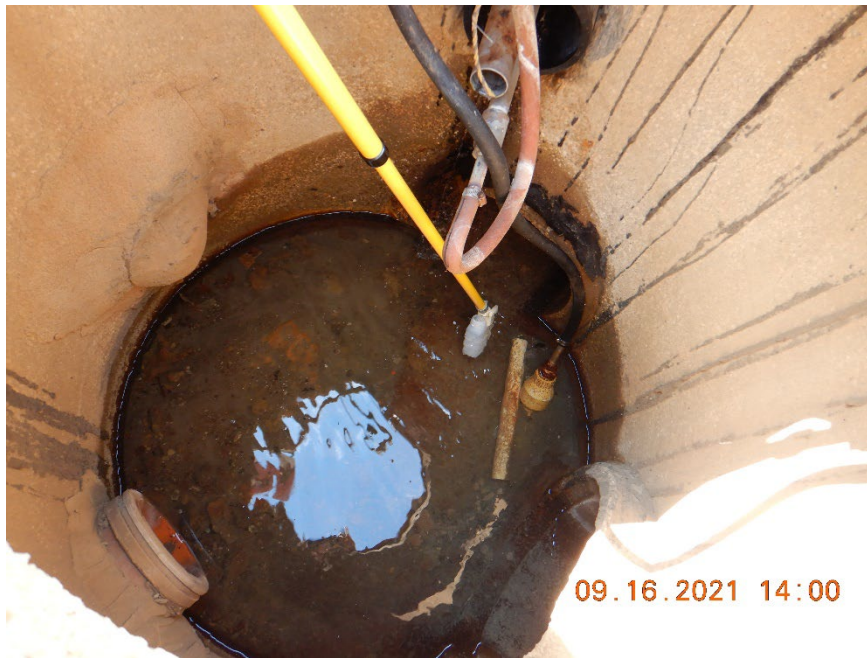
CWA Photo 33. View of sampling from the K1 process sewer.
