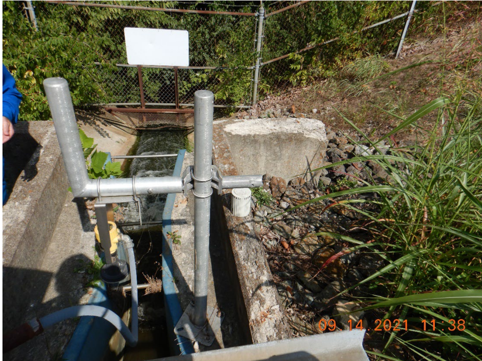
CWA Photo 19. View of the Outfall 001 flume, through which there was consistent discharge at the time of the inspection.
