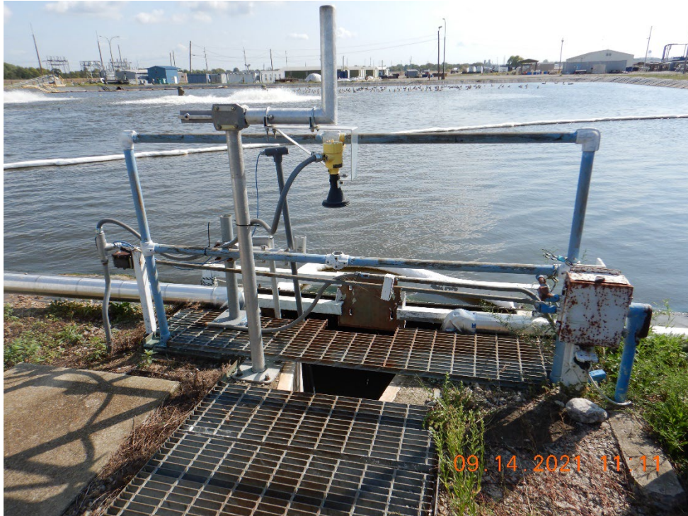
CWA Photo 15. View of the Outfall 602 flume, through which there was a consistent discharge from the South Lagoon at the time of the inspection.
