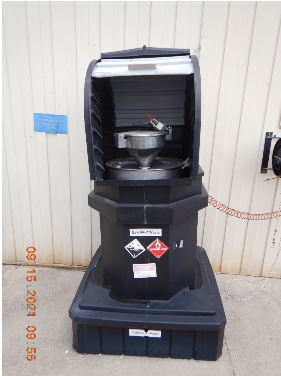
RCRA Photo 28. A view of SAA Z located on the south pad next to the facility's PAD unit. The SAA is used to manage the facility's laboratory wastes which are generated directly inside the building shown in the photograph.
