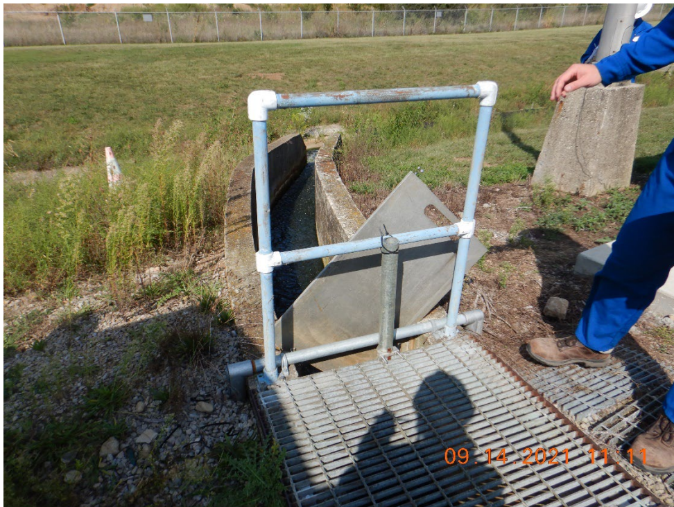
CWA Photo 16. View downstream of the Outfall 602 flume, which leads to Outfall 001.
