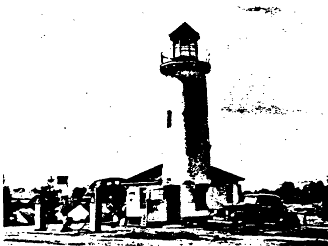
Towering concrete lighthouses were typical of the gingerbread era of service station design.
