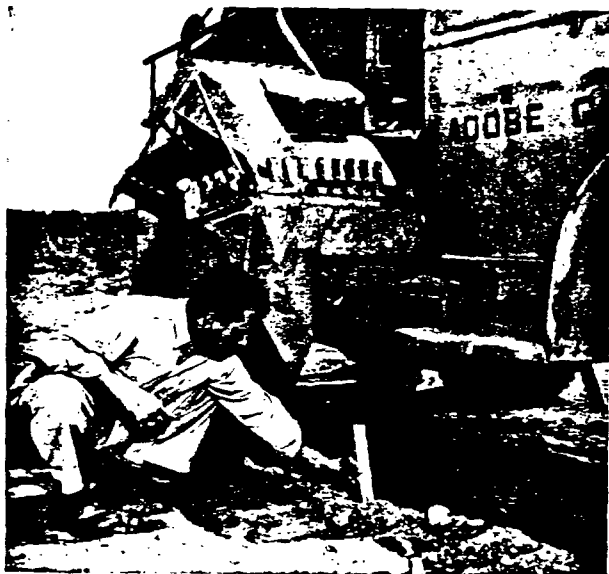
Left, a brick making machine's digging wheel cuts raw material from the earth's surface . . . Below, stabilized adobe brick is a good insulator and withstands cyclones, earthquakes and tornados.
