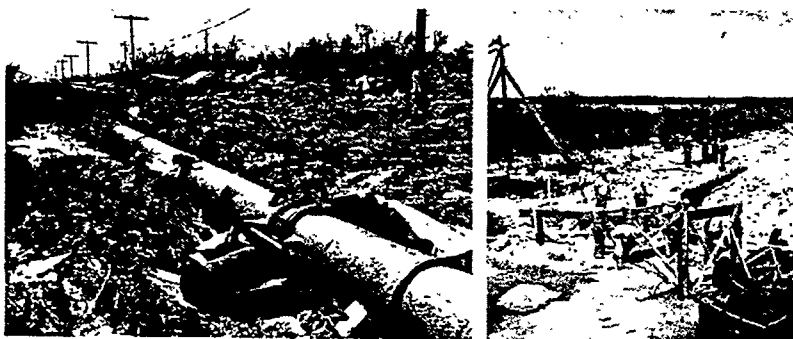
WATER LINE to Florida Keys was repaired in four days following Hurricane Donna, the Nation's first "billion dollar storm." Even before the storm had run its course, machinery was set in motion to repair the 125-mile water line extending from the pumping station in Homestead, Fla., to the tip of the badly battered Florida Keys. Setting emergency plans into action, the US Navy dispatched a plane to the Bradford, Pa., plant of Dresser Manufacturing Division, where the company supplied 100 16-inch water-line couplings for air lift into Miami. Photos show, left, how only the more exposed sections of pipeline were destroyed; right, workmen clear away debris prior to installation of new section of pipe.
