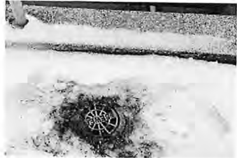
Primary Settling Tank #3 Drain Valve
