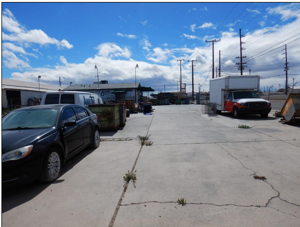
Photograph 9. View, facing south, of the Facility's impervious surface.
