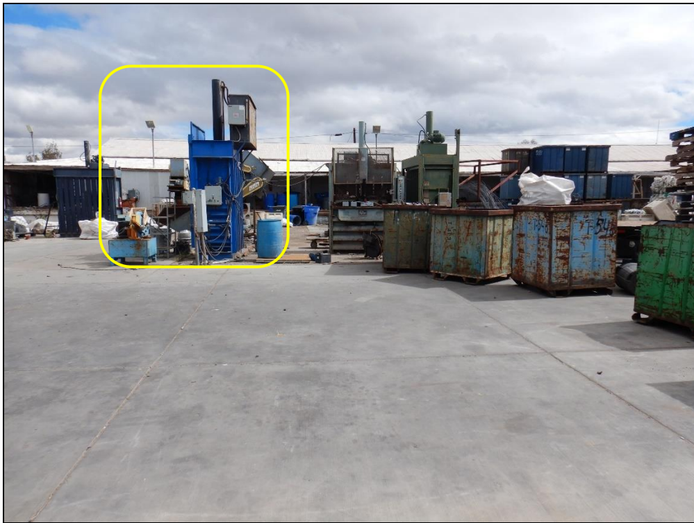
Photograph 4. View, facing east, of the Facility's machine to process materials and materials storage.
