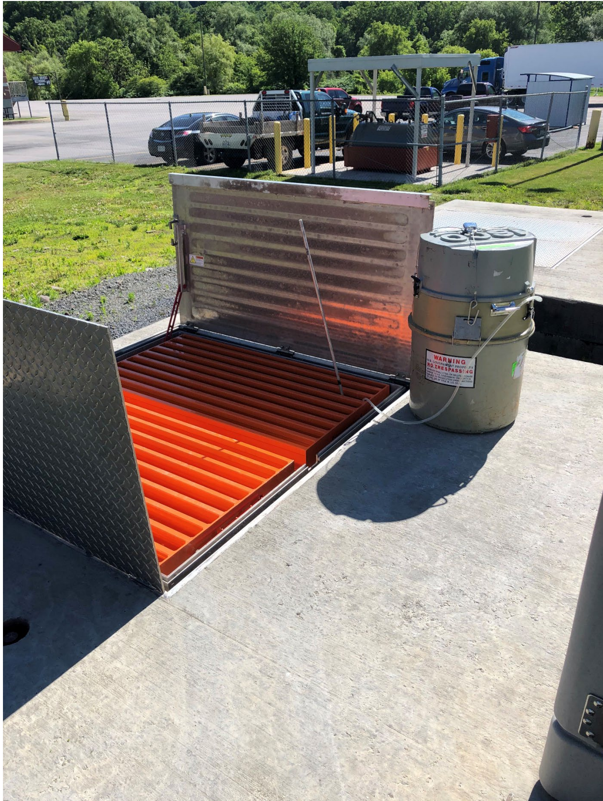
Photo #1: View of the pretreatment discharge location where samples were collected.
