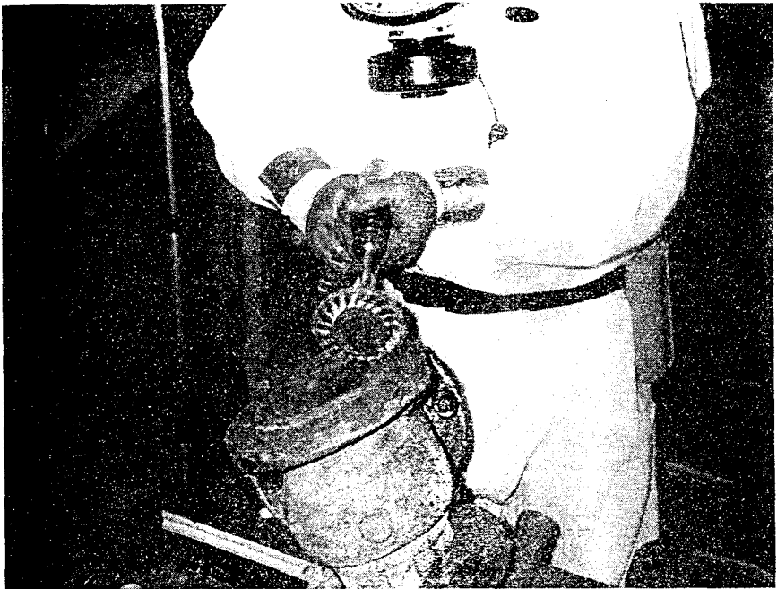
Figure 6-21. Power wire brushing of a pipe flange after the removal of the gasket during Study 1.
