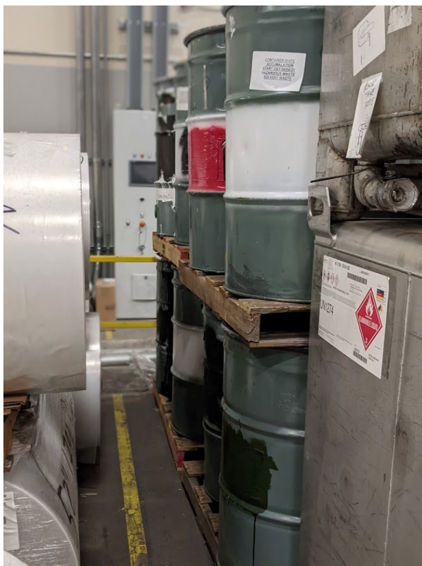
Photograph 1 of 21: Plate Mounting, Film Production Floor - Hazardous Waste CAA
