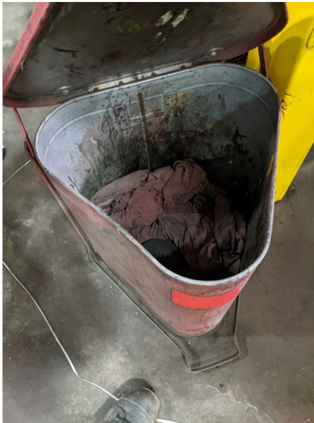
Photograph 13 of 21: Maintenance Department – Spent Rag Collection Container
