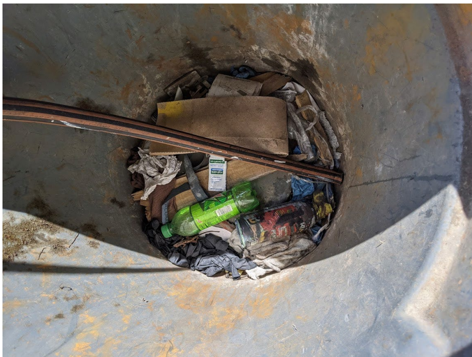
Photograph 12 of 21: Maintenance Department – Aerosol Can Disposal
