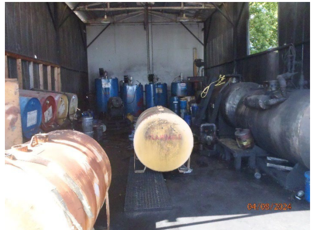
Picture 62 – Building 177 Maintenance Department used oil area
