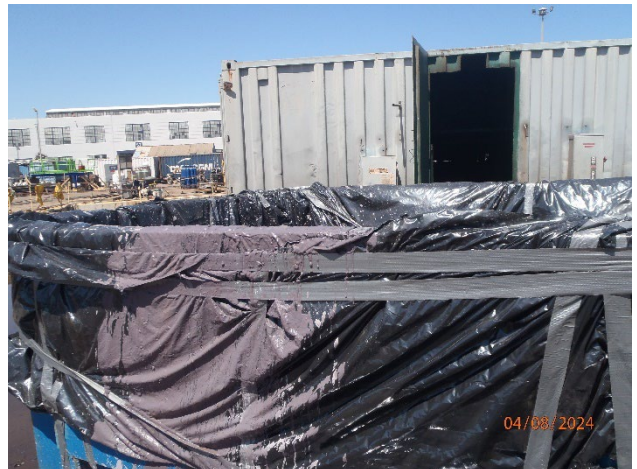
Picture 41 – Behind Condos 20-cubic yard roll-off of paint chips water slurry
