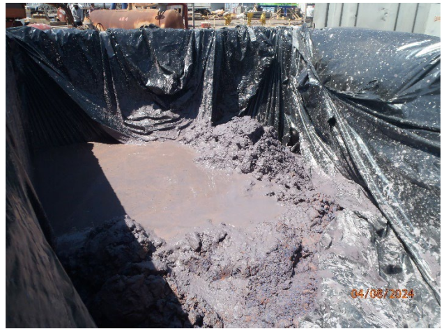
Picture 39 – Behind Condos 20-cubic yard roll-off of paint chips water slurry
