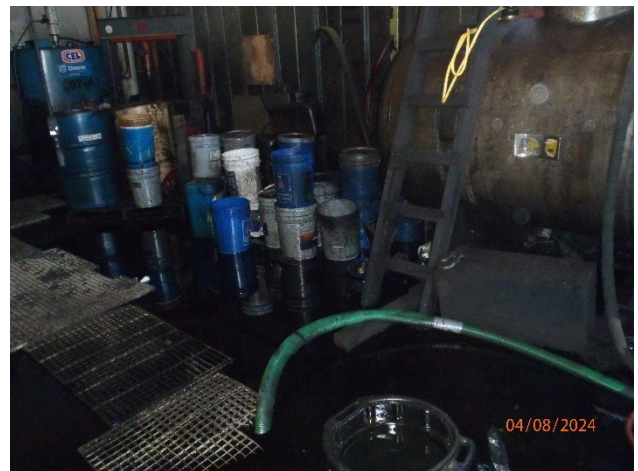
Picture 63 – Building 177 Maintenance Department used oil release to ground
