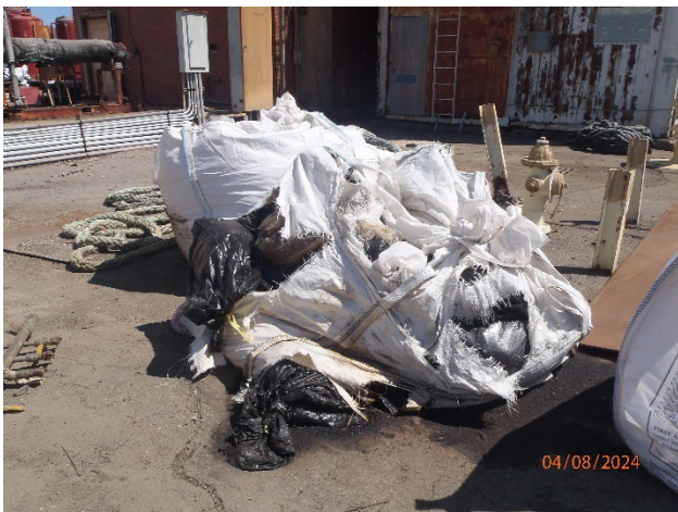
Picture 32 – Dry Dock 2 torn supersack of oily material
