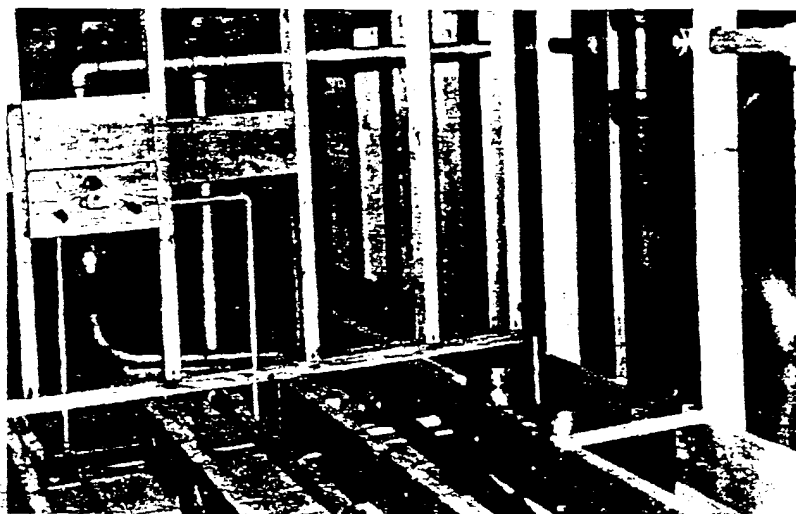
The plumbing roughing-in for Cape Cod type homes in Canton, Ohio, includes lead connections for all fixtures. Below, the lead P-trap for the bathtub.
