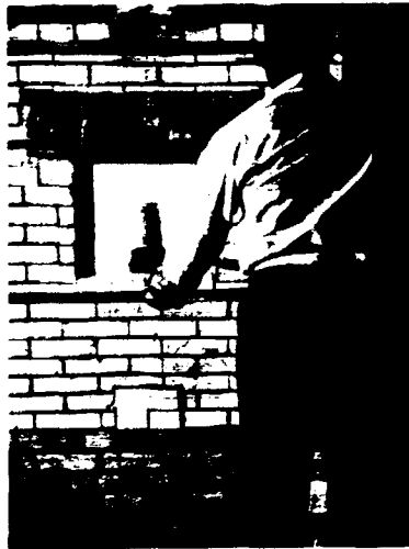
Refractory materials for lining glass and steel furnaces are test-fired at the new research lab of The Chas. Taylor's Sons Company.
