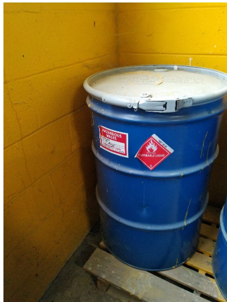
Photo 7: 55-gallon Hazardous waste SAA container near Coal Tar Line.
