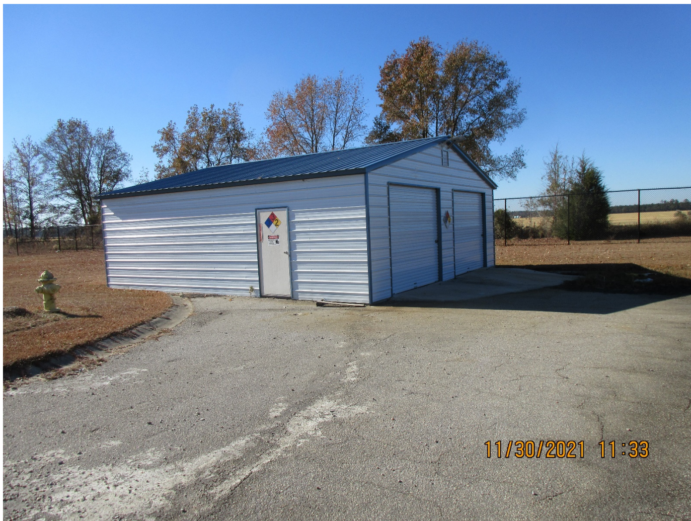
Photo 18 – Facility’s 90-day Hazardous Waste Accumulation Building
