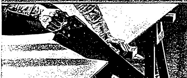
Recessed-Edge Sheetrock is cut to size by scoring with a knife or chisel and breaking or sawing with a sharp hand saw.
