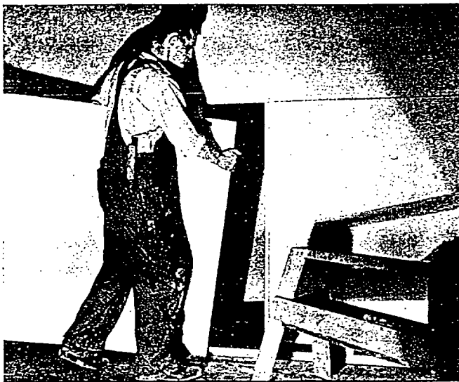
Recessed-Edge Sheetrock being applied horizontally—at right angles to framing—to give increased bracing strength.
