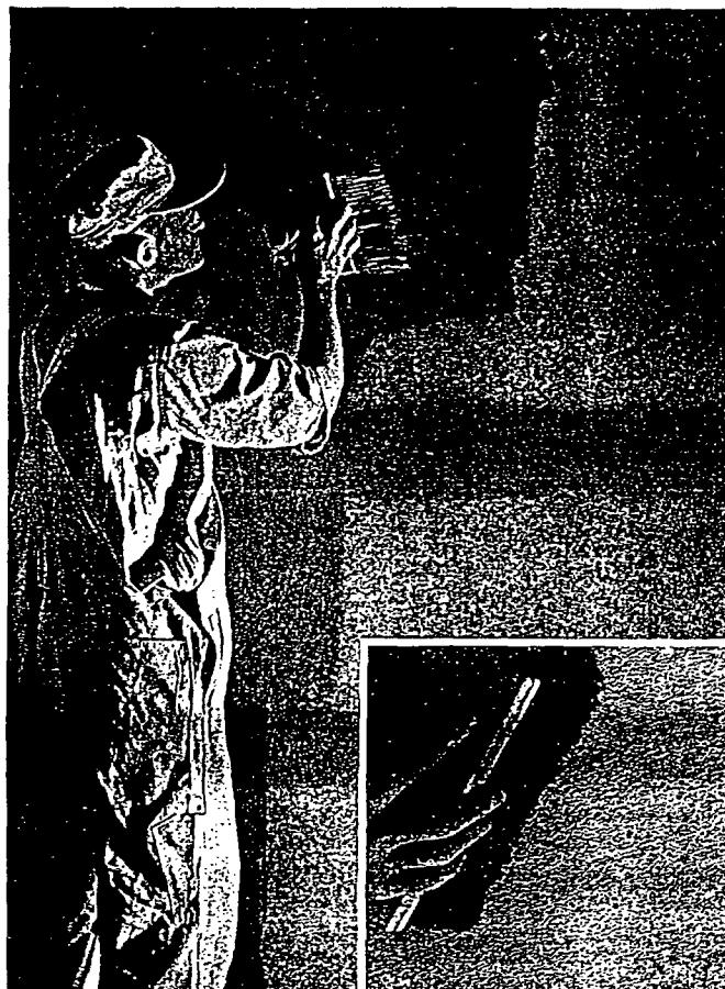
(Above) Textone being applied over Recessed-Edge Sheetrock—Perf-A-Tape wall. Insert shows how fine Colonial stippled effect is obtained. (Below) The finished job—walls of Recessed-Edge Sheetrock, joints reinforced and hidden with Perf-A-Tape, decorated with Textone and Texolite.
