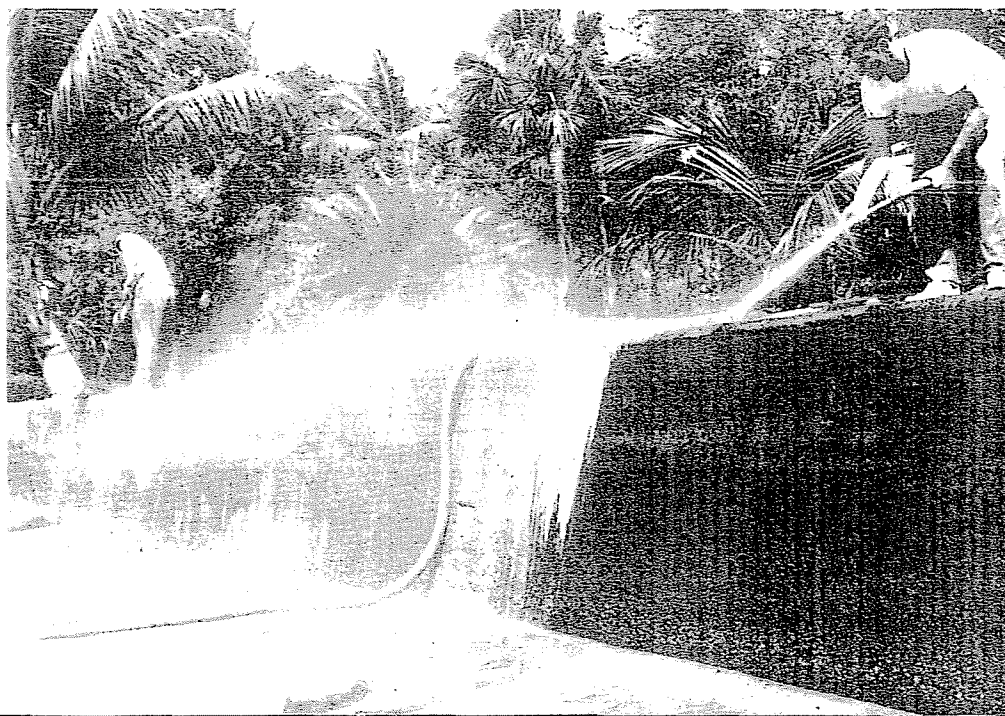
A striking after-and-before view of a fuel oil coated sea wall being cleaned by hosing (40 lbs. pressure) with sea water after spraying on a heavy-duty marine cleaner.
