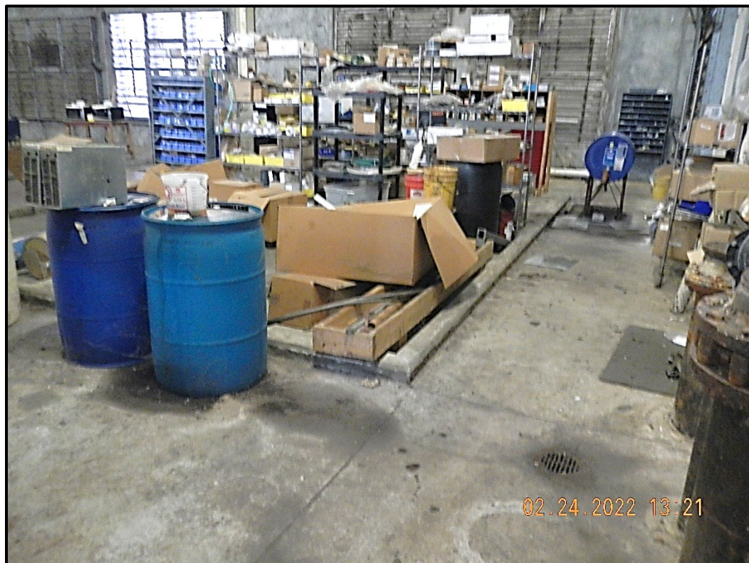
Figure 15. Parts Storage and Equipment Maintenance Room – Drains Outside Berm
