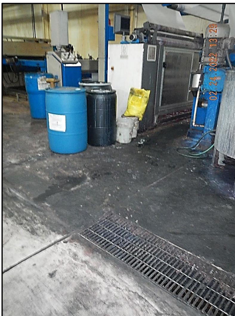
Figure 13. Additional Chemicals In Use Lacking Secondary Containment
