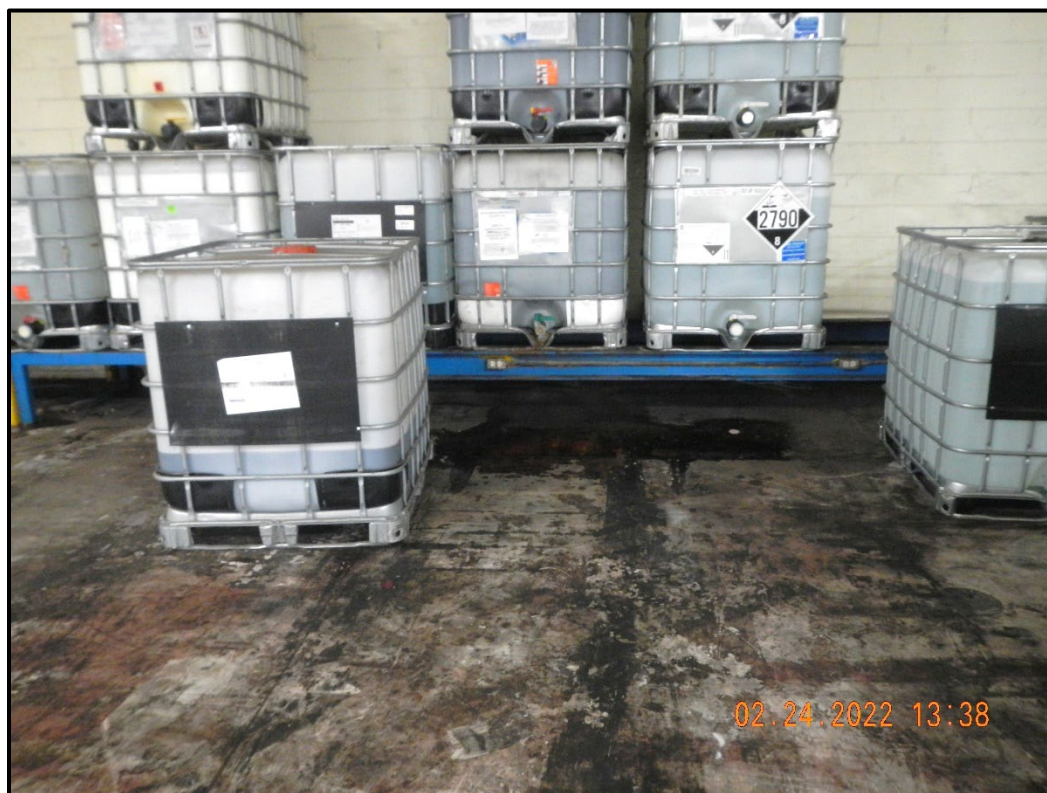
Figure 17. Un-bermed Bulk Chemical Storage Area – Spillage Under Rack
