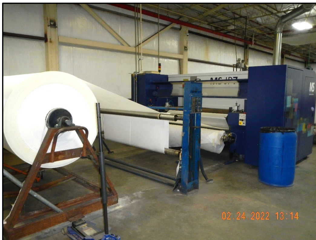
Figure 7. Digital Printing System in Production Area
