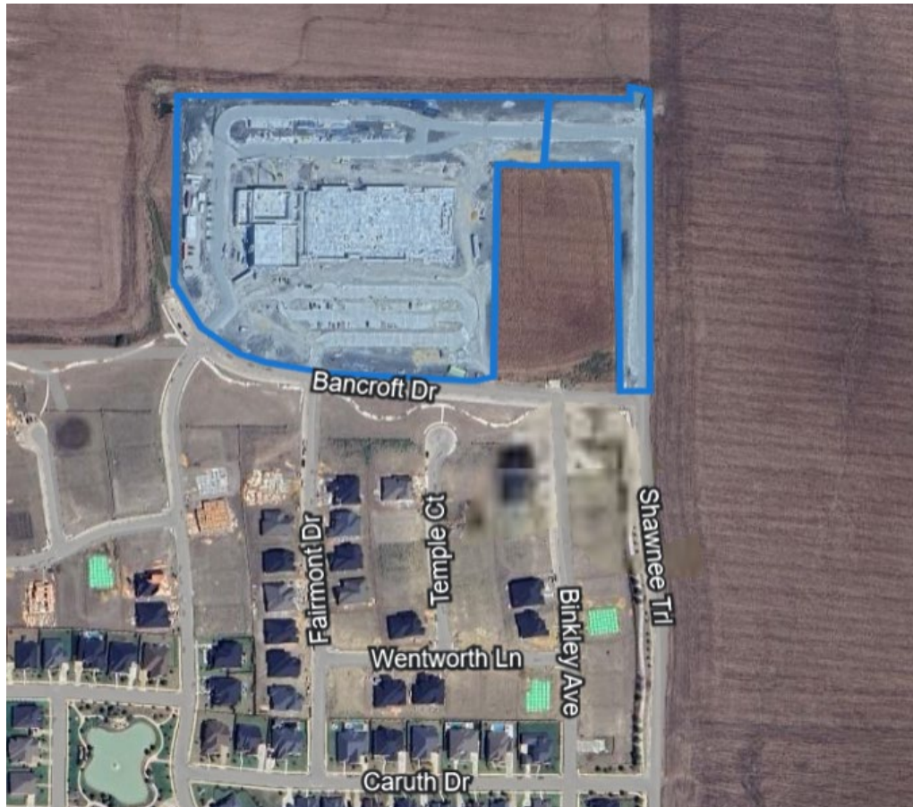
Aerial Image 1: The New Elementary School #19 commercial construction site. The site is located within the approximate blue boundary lines depicted above (northwest of Shawnee Trail and Caruth Drive).
