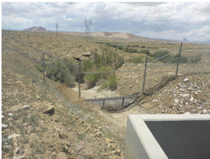
Photo 5 : Looking downstream from Outfall 001 towards No-Name Wash.
