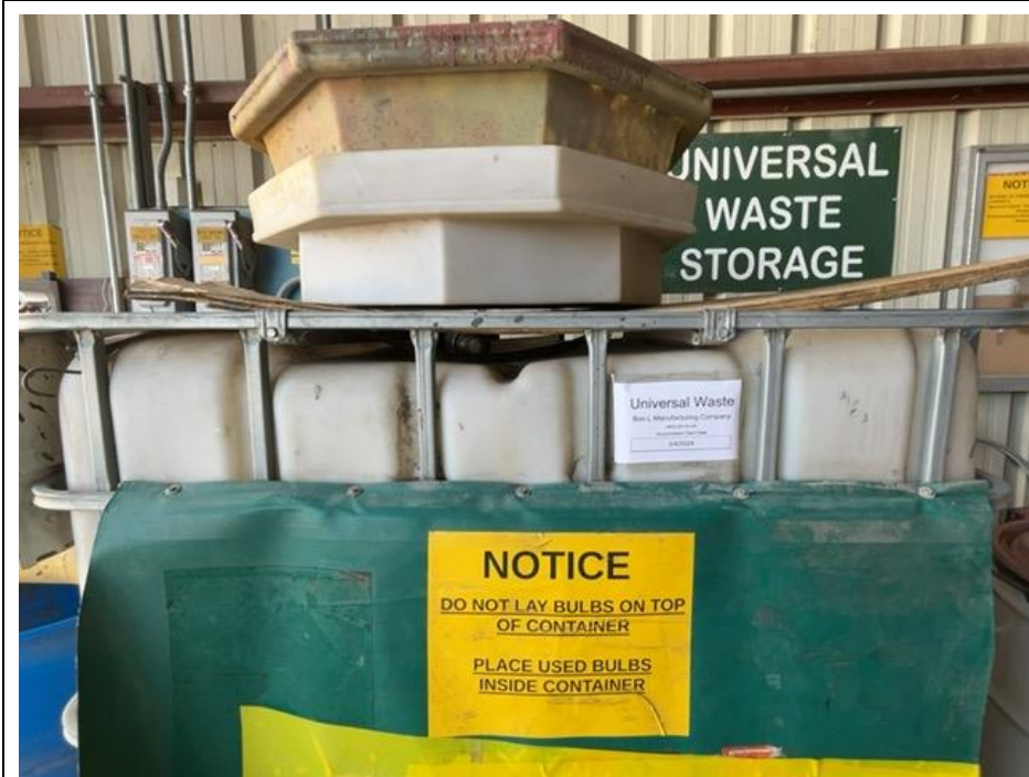
Photo 21 – Tote for Universal Waste Lamps in CAA
