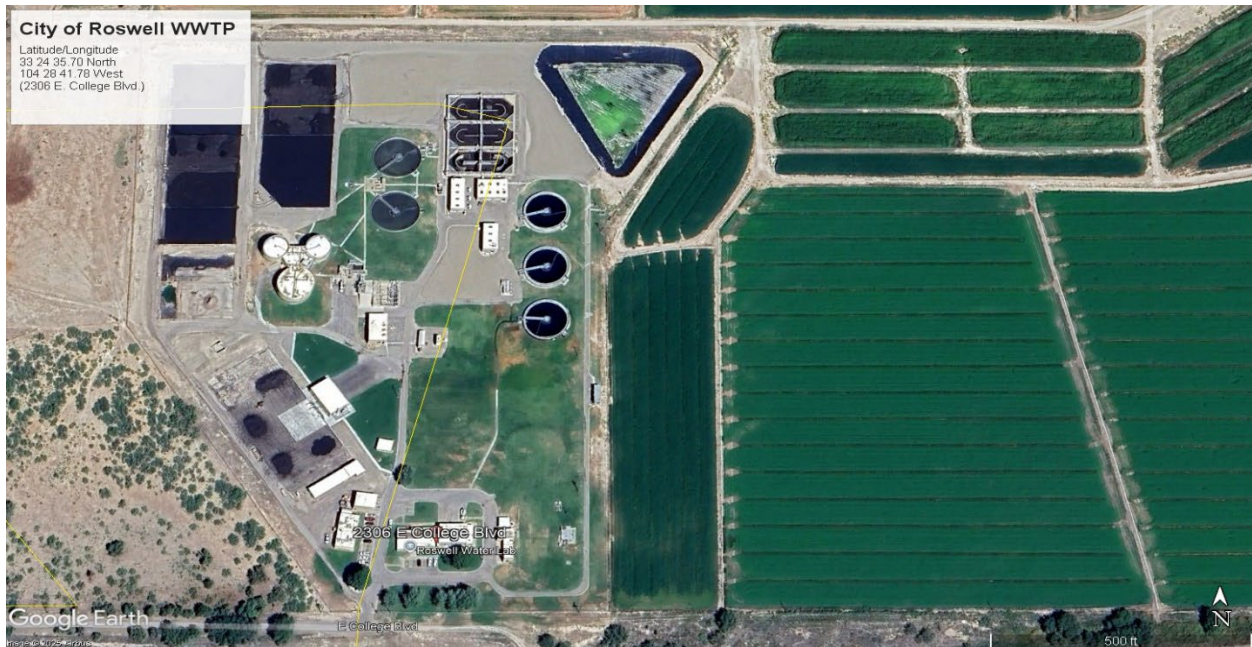
Aerial Image #1: Overall view of the City of Roswell’s Wastewater Treatment Plant. Aerial from Google Earth maps.
