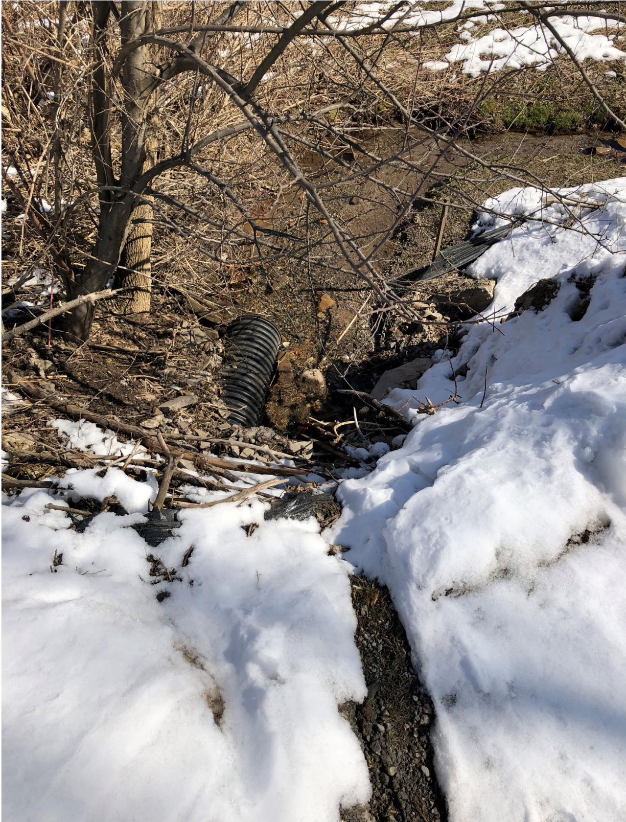
Photo #3: View of stormwater Outfall 003.
