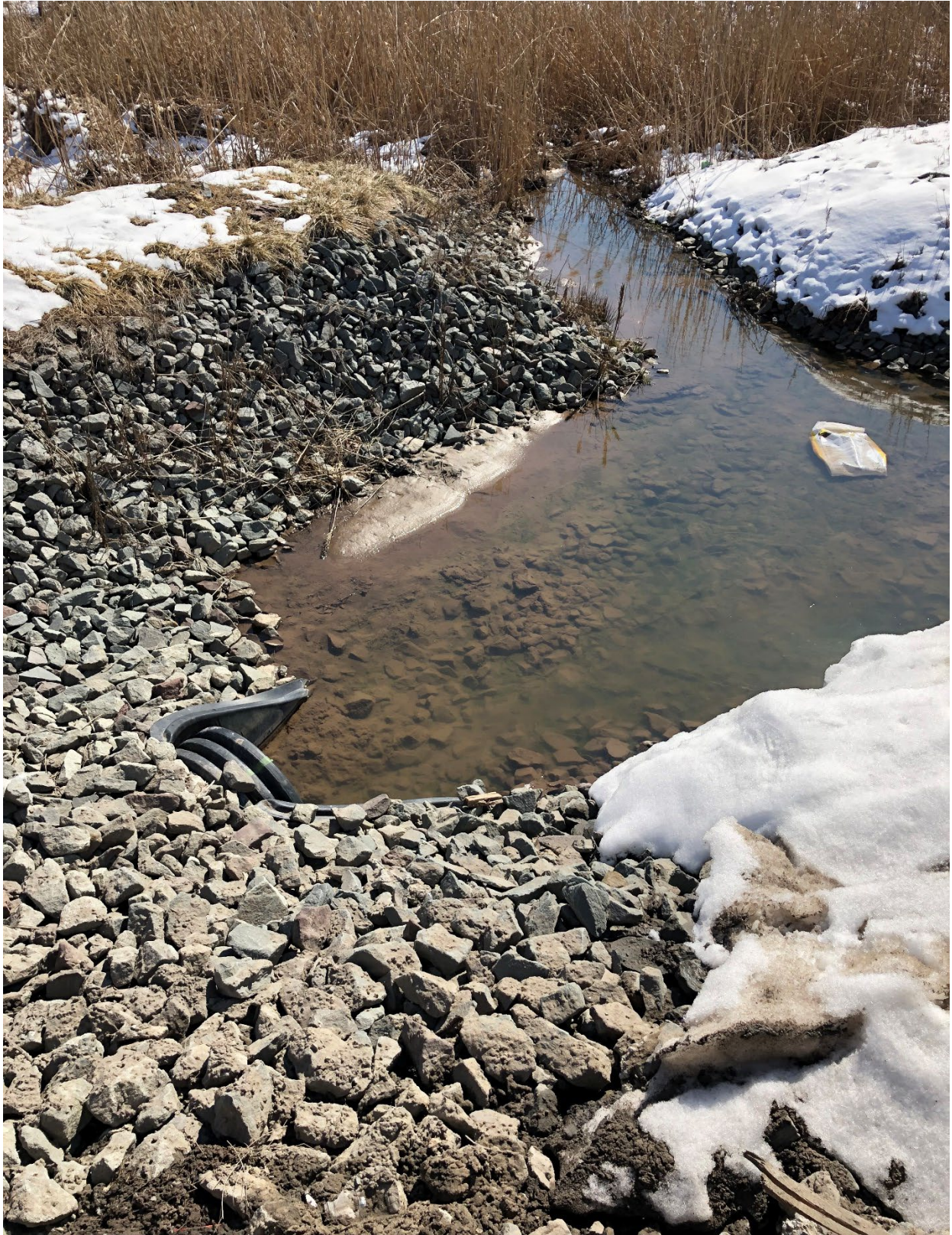
Photo #2: View of stormwater Outfall 002.
