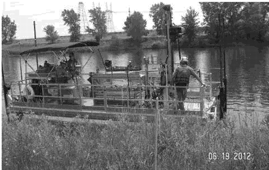
Sonic rig used to install sampling wells
