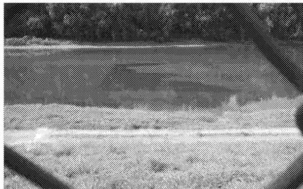
CCS cap filling with clean river sediment which naturally moved down the river system.
