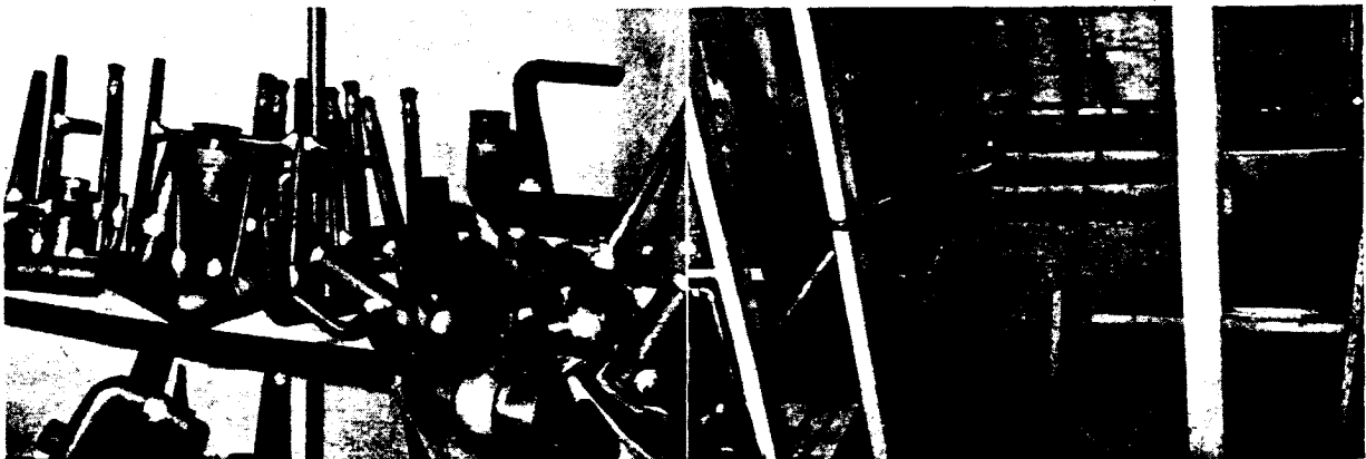
At left, some of the lead frames ready for installation in the remodeled Missoula Hotel, Missoula, Mont., and at right, small-home lead roughing following the principles of Stamford's Double-Lifetime Home
