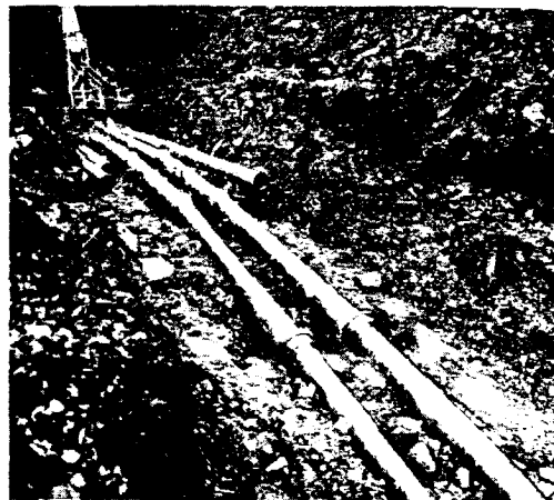
At left, a view of the 8-in. effluent pipe line and, at right, 8-in. effluent, influent and overflow lines for the new Cincinnati control reservoir
