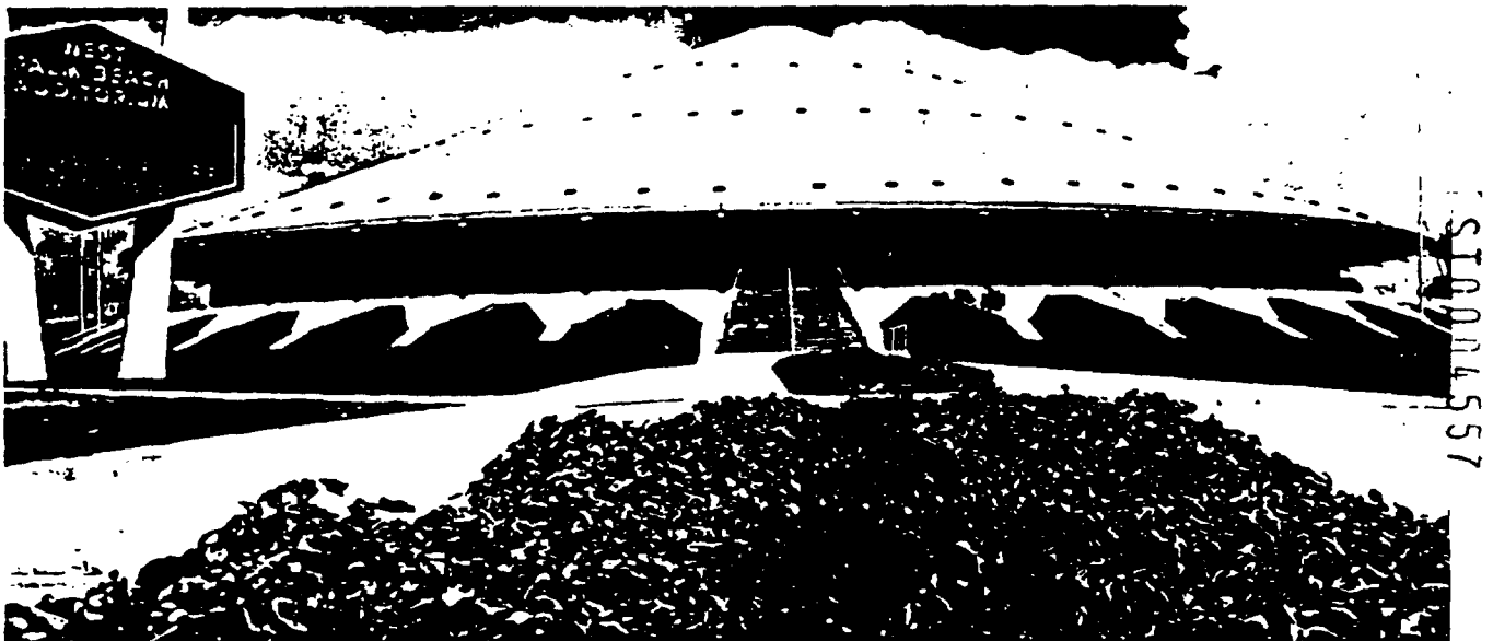
Chlorinated polyethylene from Dow is incorporated in Celotex Corporation's single-ply roof membrane for West Palm Beach Auditorium.
