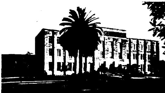
The Hancock Foundation Building, University of Southern California, uses lead pipe and valves for salt water lines
