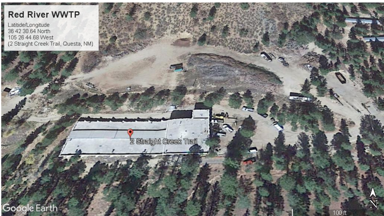
Aerial Image #1: Overall view of the Town of Red River’s Wastewater Treatment Plant. Aerial from Google Earth maps.
