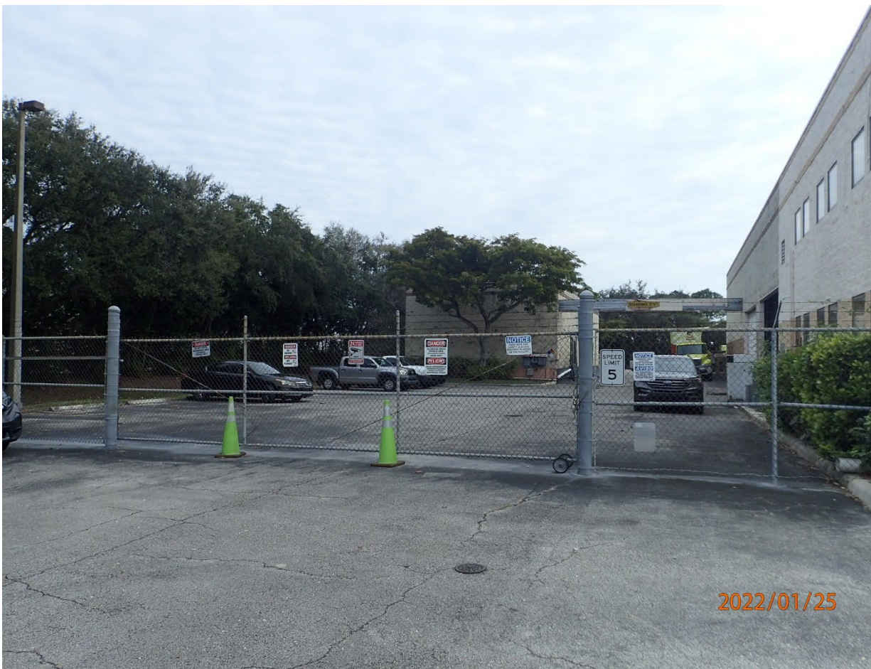
Photo 1: Front gate secured with Danger signs.
