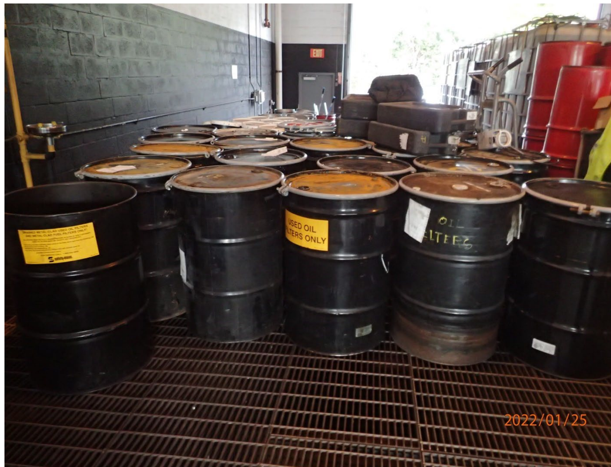
Photo 7: Non-hazardous waste container storage (used oil and used oil filters).
