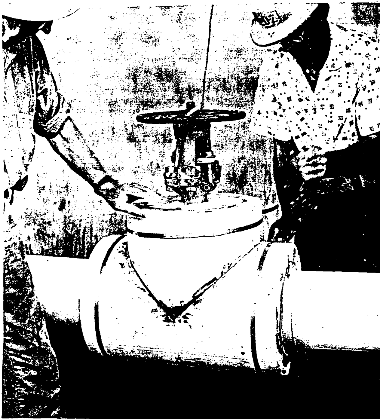
Flanged Globe Valve Cover Secured In Position
